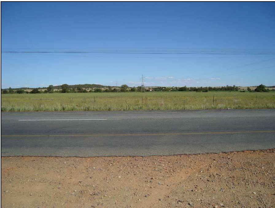
Fig.21 Point 19. Power line crossing N12.
