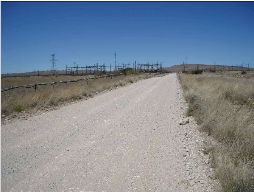
Fig.1 Garona Sub-Station near Groblershoop (Point 1 Map 9).
