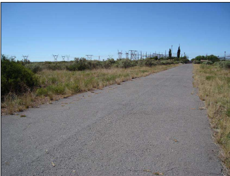
Fig.7 Point 12. Ferrum Sub-Station at Kathu.
