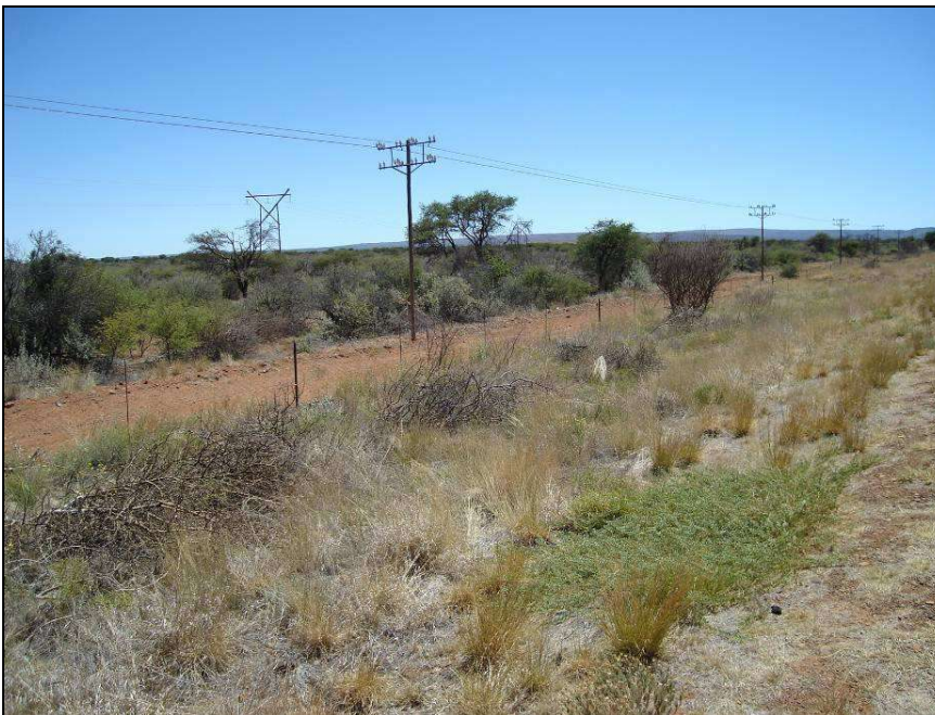
Fig.15 Point 7. Power line crossing the N14.
