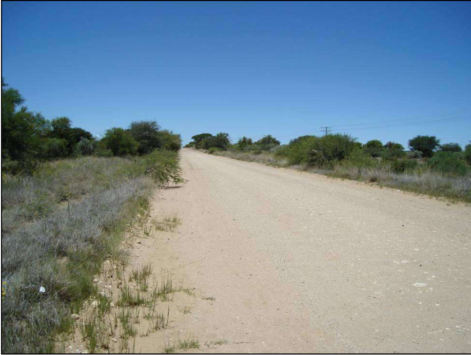
Fig.18 Point 14. Power line to cross the R371 road to Lykso.
