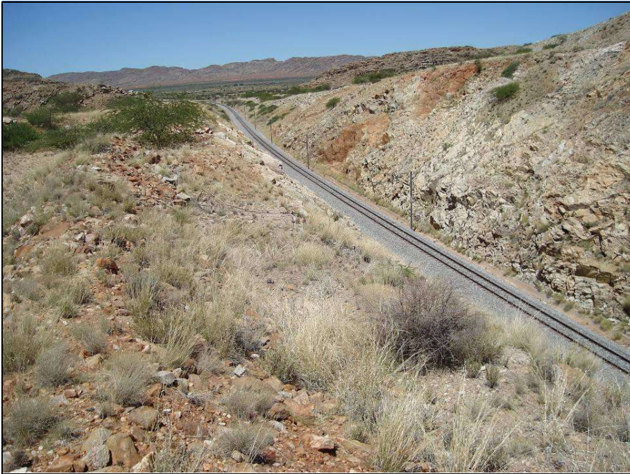
Fig.2 Point 2. The cutting for the railway line.
