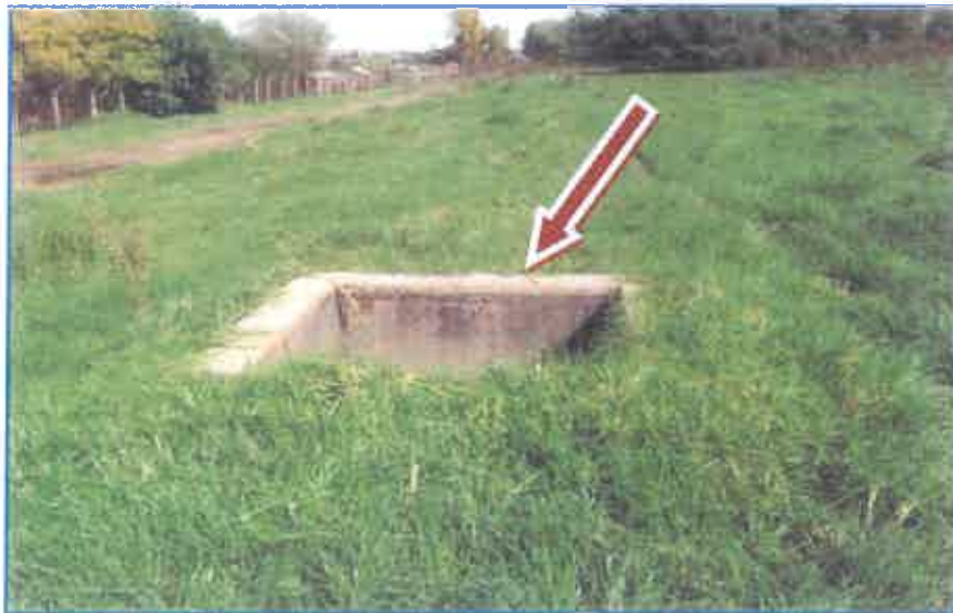
Figure 2: View of the existing concrete Manhole of the sewage pipe line
