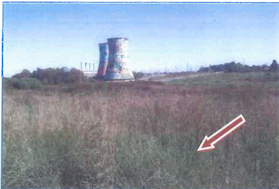
Figure 10: View of the proposed site D located adjacent to Orlando cooling tower, the area is located north of the Bara Mall.
