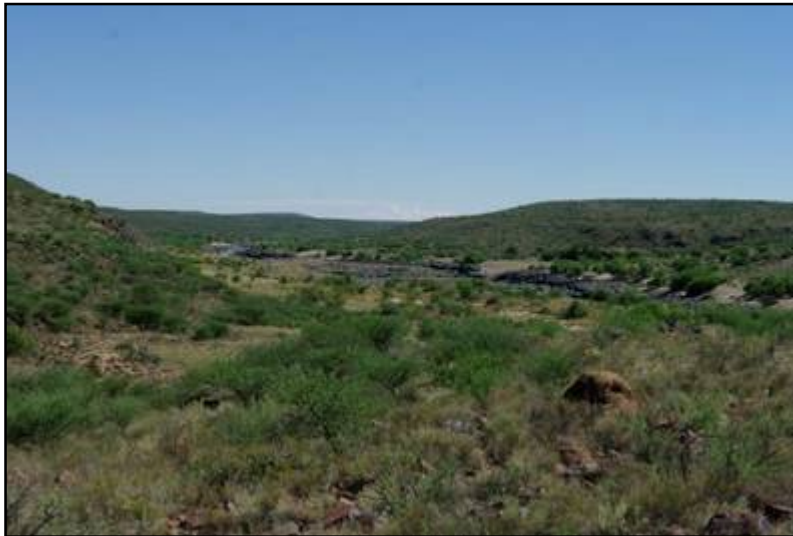
Plate 114: General view of the Rooikat Hydroelectric Power Site from the south bank
