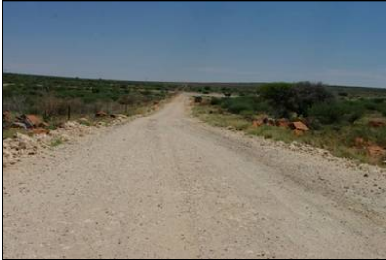
Plate 128: General view of the Alternative Construction Road [1]
