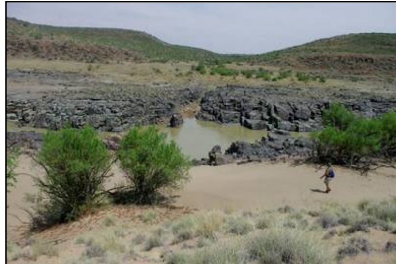
Plate 115: General view of the Rooikat Hydroelectric Power Site from the north bank
