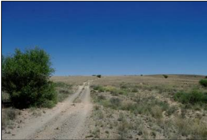
Plate 121: General view of the South Access Road [2]
