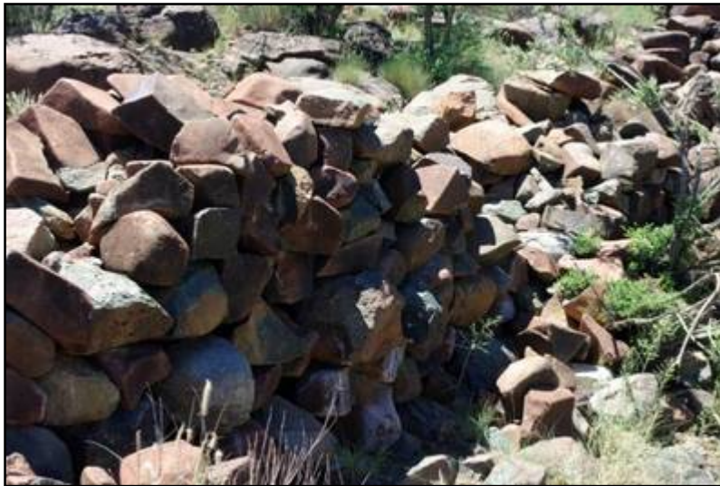
Plate 16: Close-up of wall remains at RH-05.1
