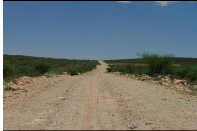
Plate 130: General view of the Alternative Construction Road [2]
