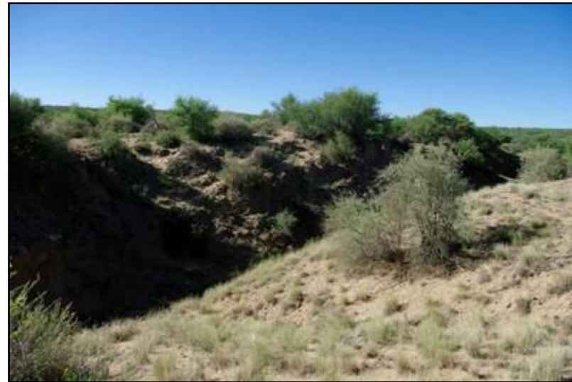
Plate 123: View of the South Access Road in the vicinity of the weir
