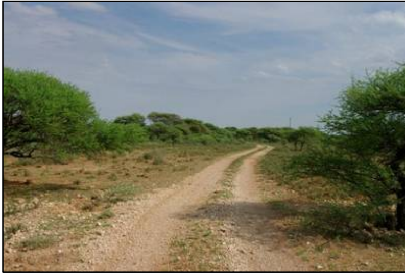
Plate 124: General view of the North Access Road [1]
