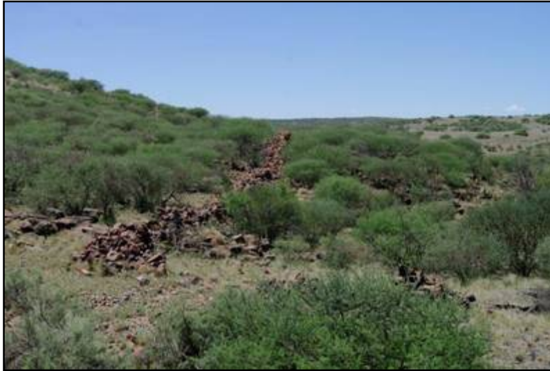
Plate 15: View of the RH-05.1 stone wall
