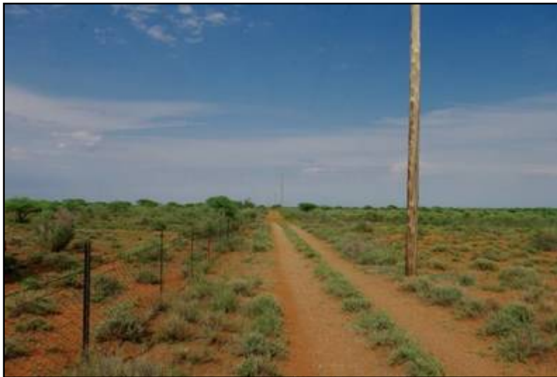
Plate 125: General view of the North Access Road [2]
