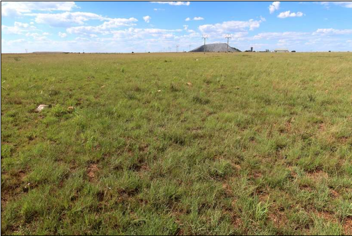
Figure 7: View north-eastwards from the solar plant project area towards the Vaal Reefs Nine 132/6.6 kV Substation adjacent to the mine seen on the skyline. The proposed grid connection will run across the intervening flat grassy terrain where bedrock exposure is very limited.
