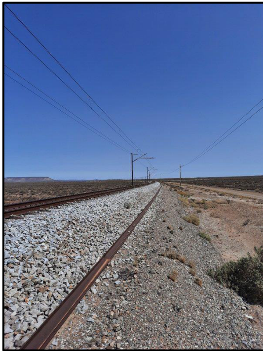
Figure 7.4. Existing railway in the study area.
