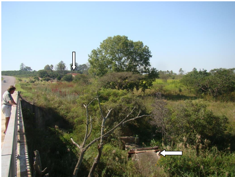
Fig. 2: A general view of the study area from the new bridge on the R40. The bridge is located on the south western corner of the study area. One of the residences is seen in the background (see arrow). The old bridge across the White River is below the new bridge (see arrow).
