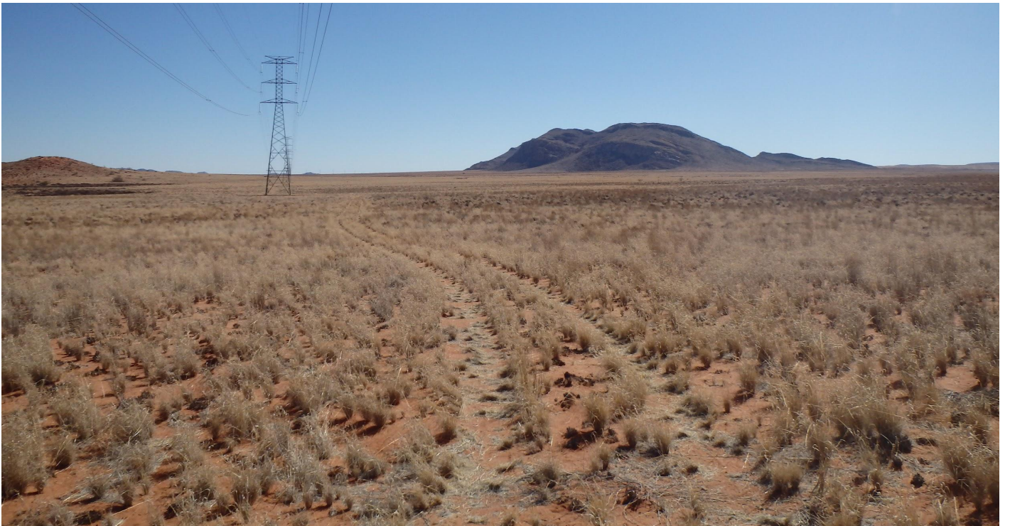
Figure 5.8 View of Swartberg and the existing ohl in the PV area.
