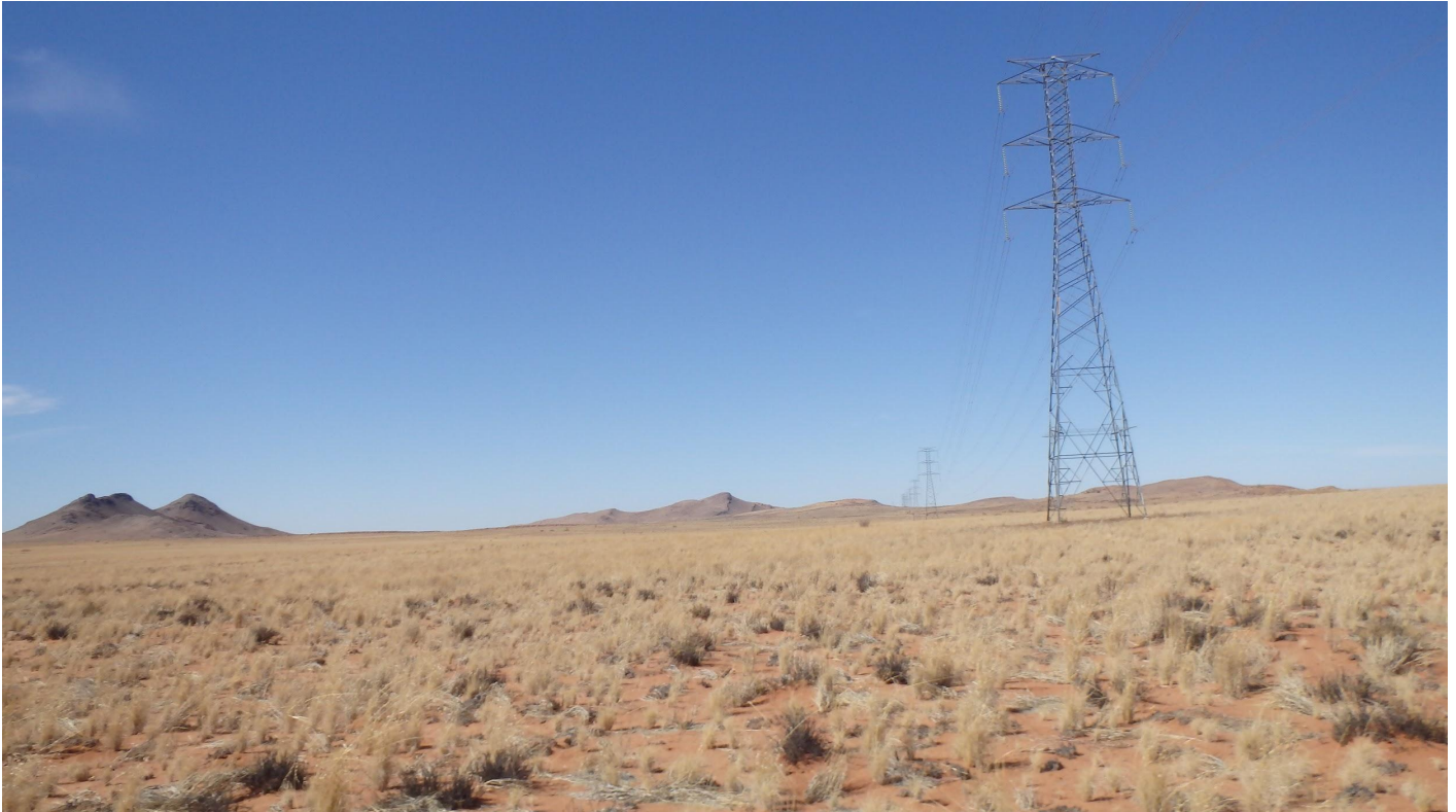
Figure 5.5 View in the PV area of the 200kV ohl, Platjiesvlei se Kop and the level plain.
