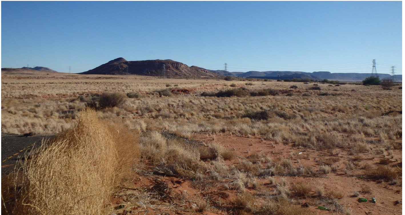
Figure 5.1 View of the 200kV overhead powerline route from the N14 highway
