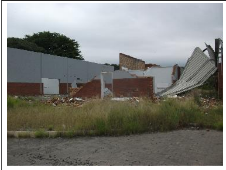
Figure 6- Demolished and abandoned mining infrastructure in the centre of the project area (above).
