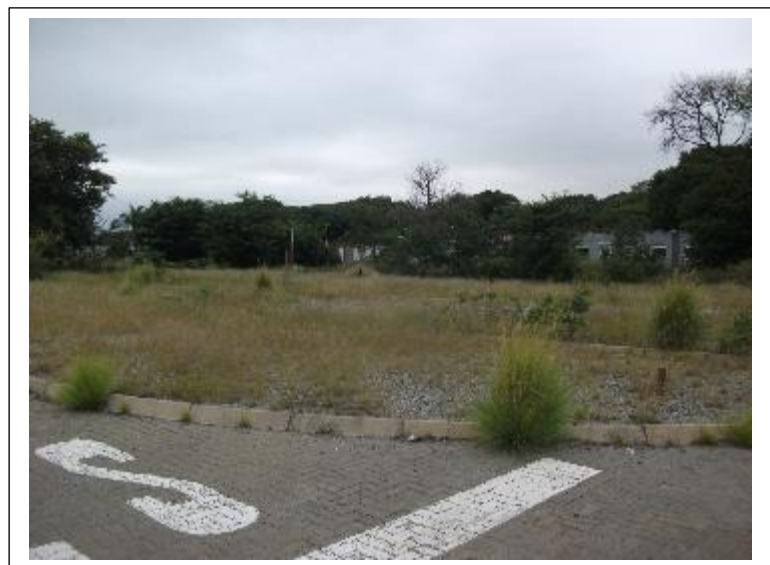
Figure 9- More demolished and abandoned mine infrastructure which covers a substantial surface area in the centre of the project area. These remains have no heritage significance (above).
