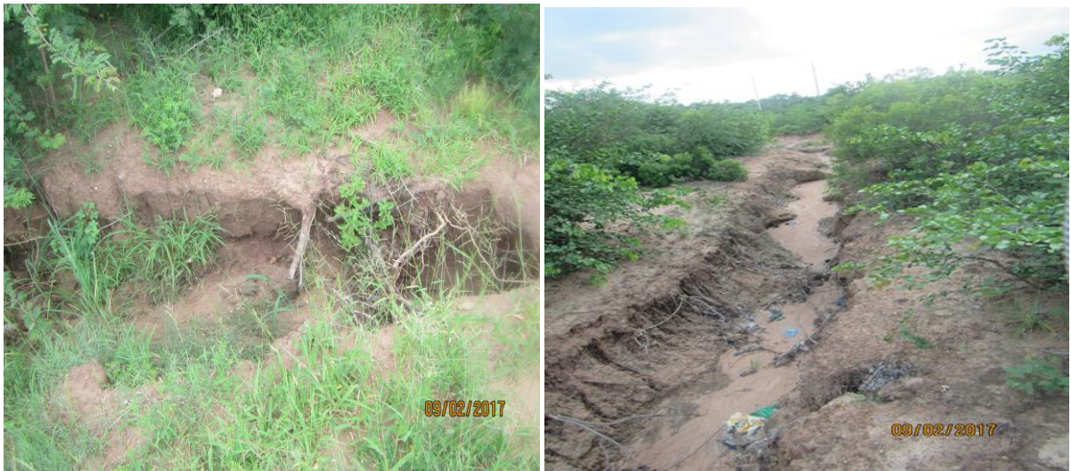
Figure 7: Some of the inspected trenches within the project servitude.
