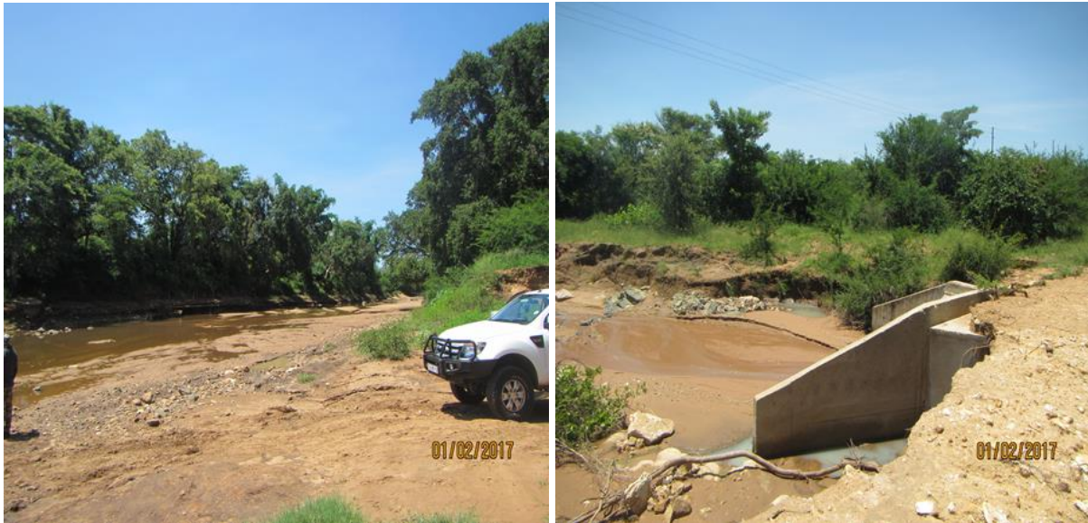
Figure 8: Some of the inspected area along the river banks.
