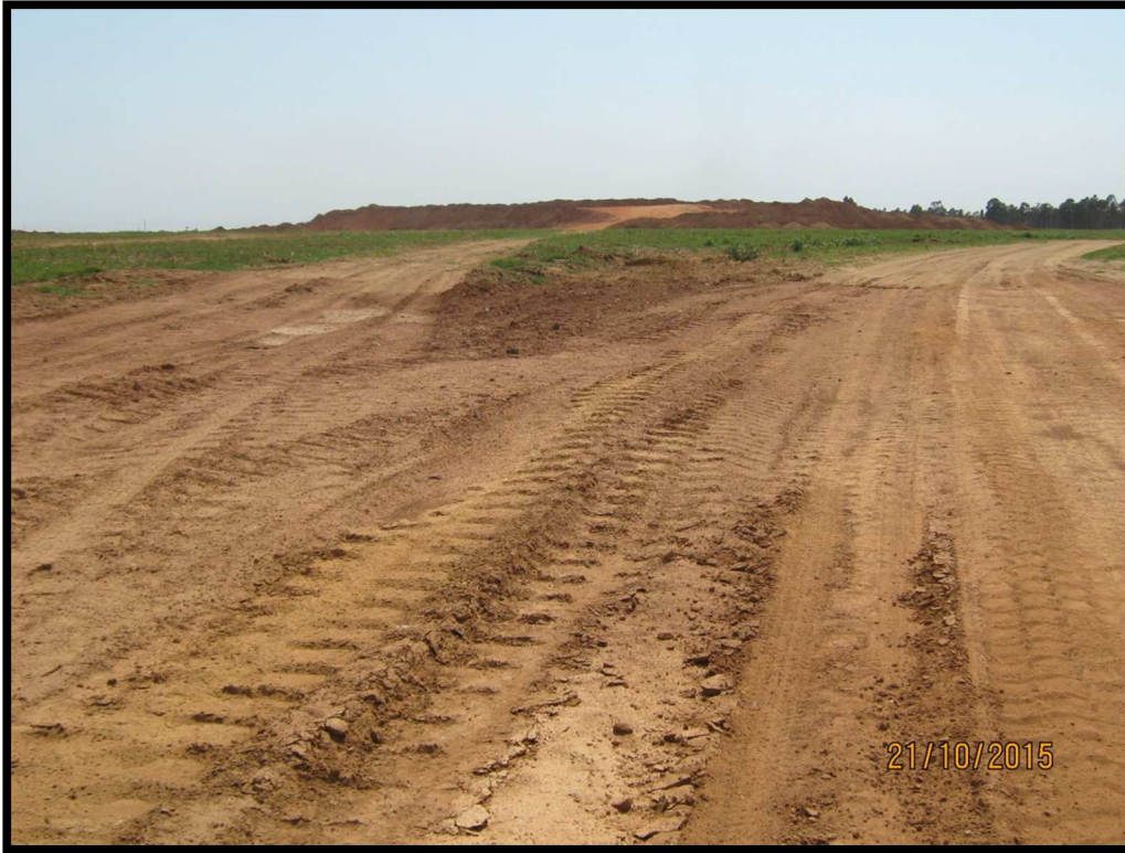
Figure 8: View towards southern section.
