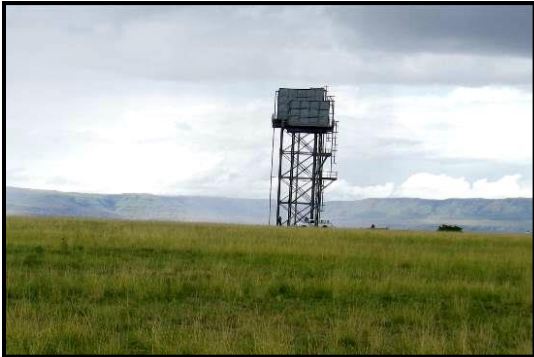
Figure 3. Photograph showing the existing water tower adjacent to the proposed powerline route. No heritage sites occur on the footprint.
