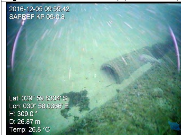
Figure 8: Concrete pipe (SAPREF 2016)
