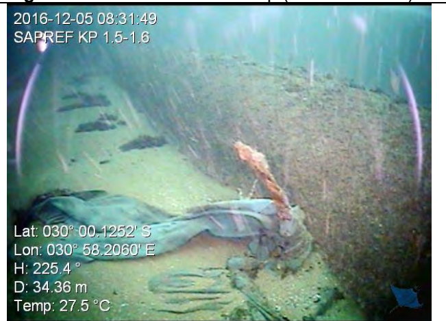
Figure 9: Steel cable with plastic attached (SAPREF 2016)
