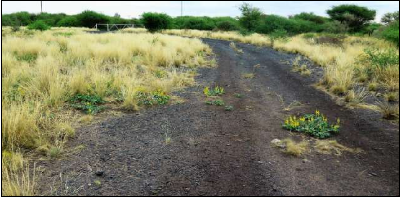
Figure 14: The BIF used to line the Eskom servitude road across the property. It litters the southern section of the study area, along the R31 and the railway line too.
