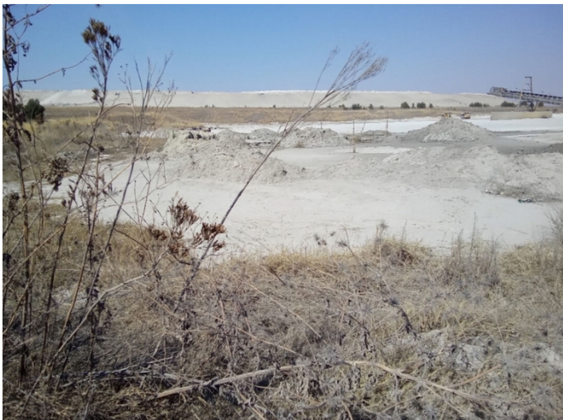
Figure 9 – View of ash dump in the background with silt storage in
