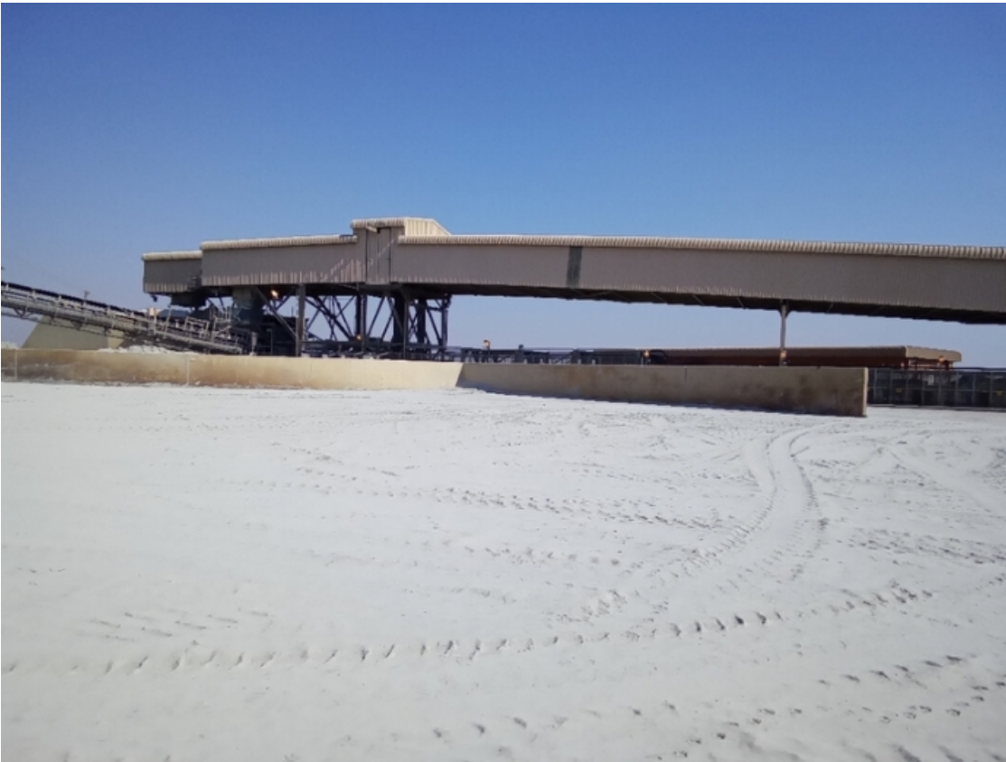
Figure 11 – Existing radial stacker and slab area (-25.928200; 28.906444)
