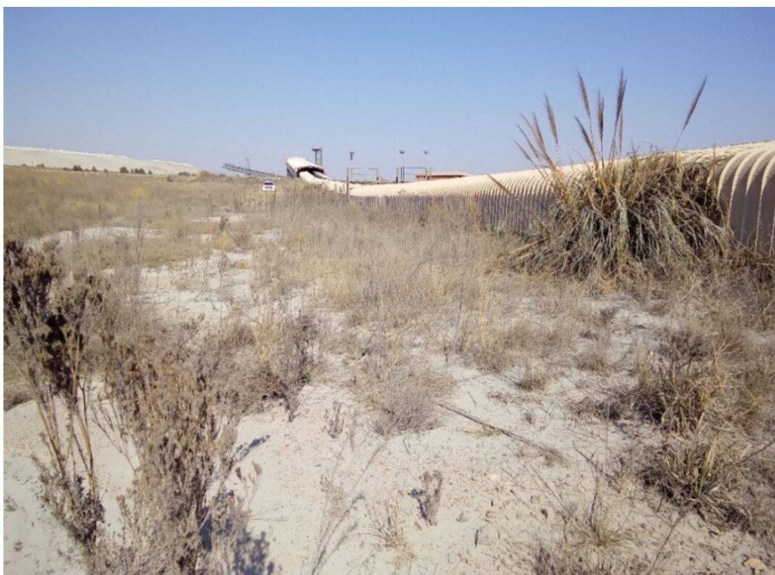
Figure 7 – Conveyor towards the radial stacker (-25.926564; 28.907850)
