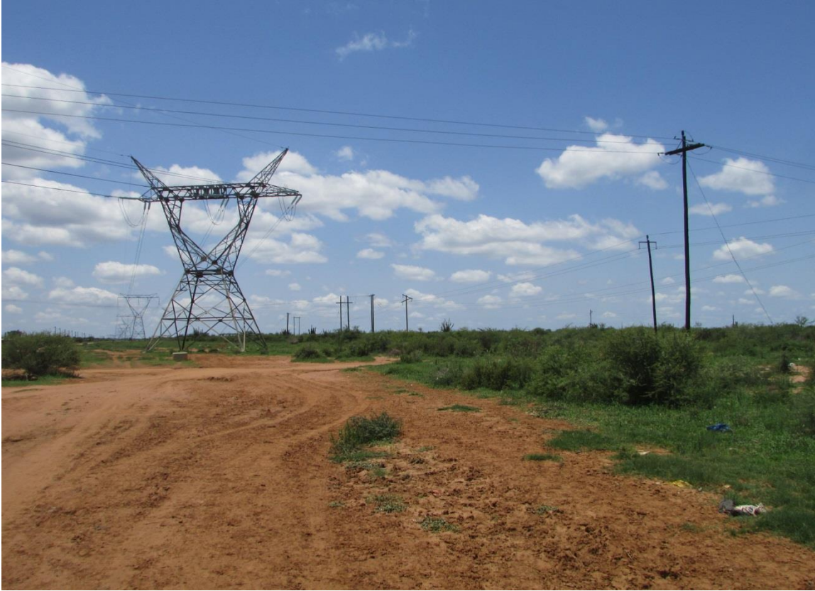
Figure 21: Another view of the existing ESKOM line that will be used.
