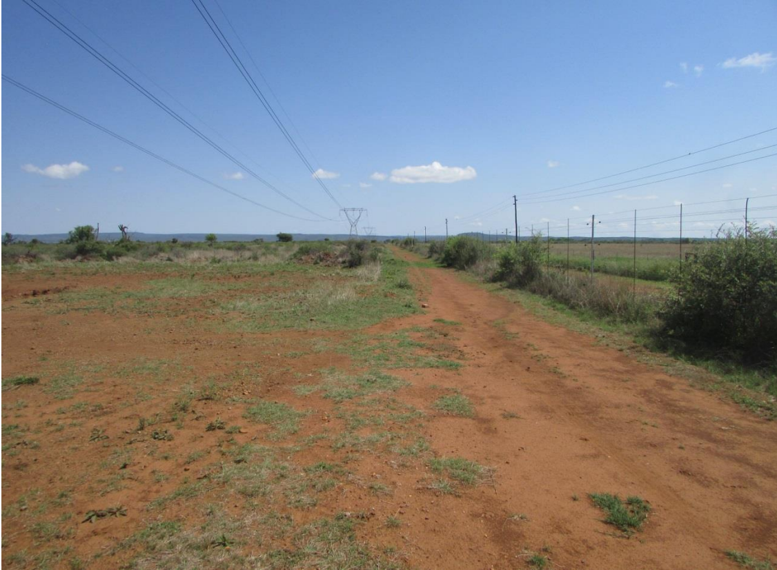
Figure 14: View of part of the existing Eskom Powerline and servitude.
