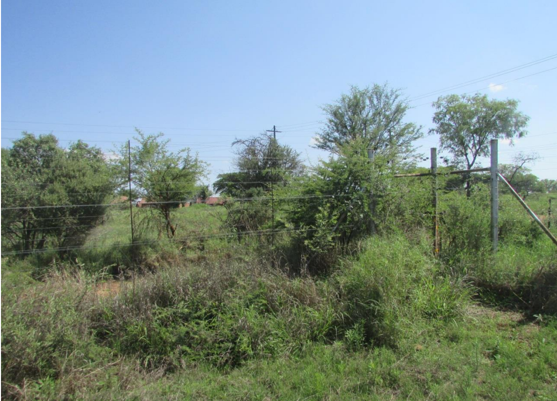
Figure 18: At the start of the Grid Connection Corridor using the existing Eskom line towards the Warmbaths Substation to the north.
