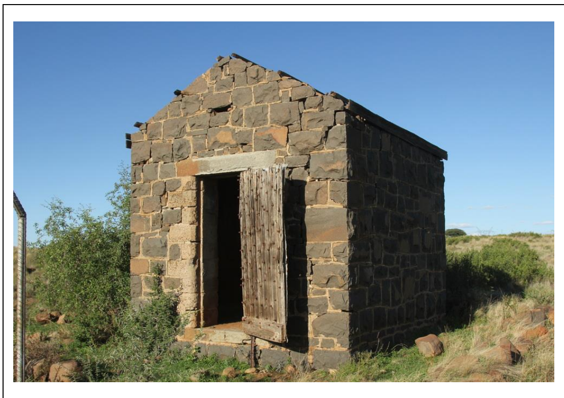
Figure 7. Old powder magazine located outside of Luckhoff, dating to the 1880s
