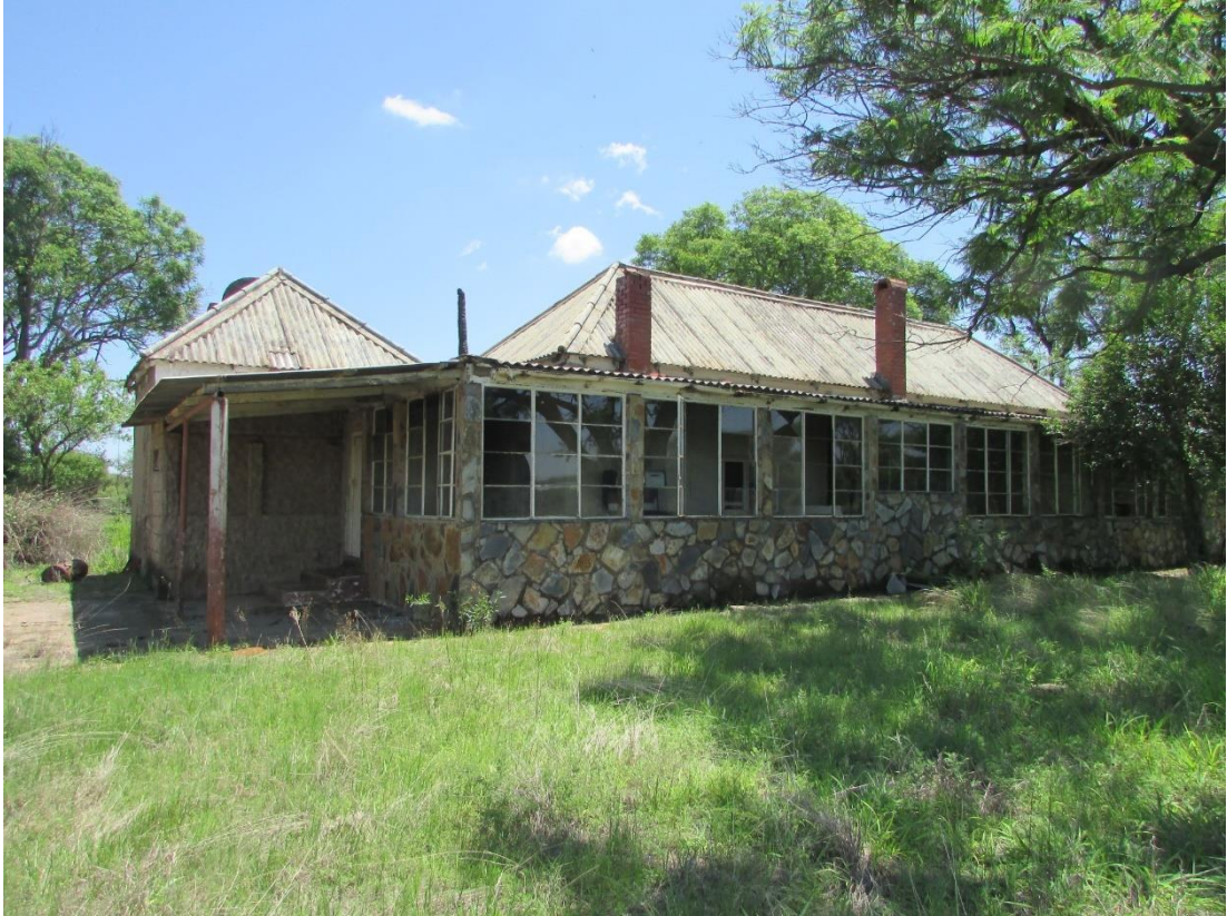
Figure 37: A front view of the main homestead on Site 7. Although there has been many alterations and additions, the original style is typical of the late 19 th /early 20 th centuries.
