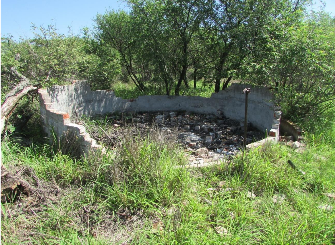
Figure 23: Remains of an old cement dam/reservoir on the site.
