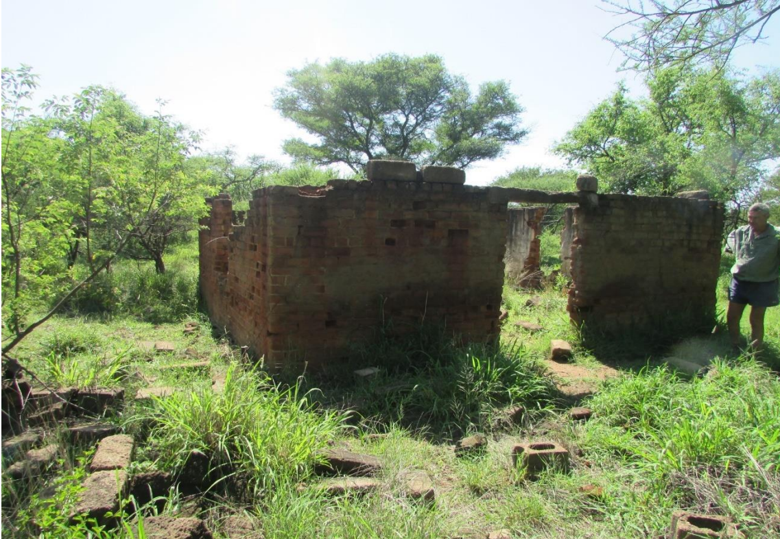
Figure 16: A view of Site 2.
