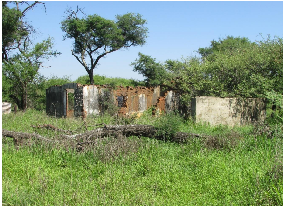
Figure 18: Another structure on the site.
