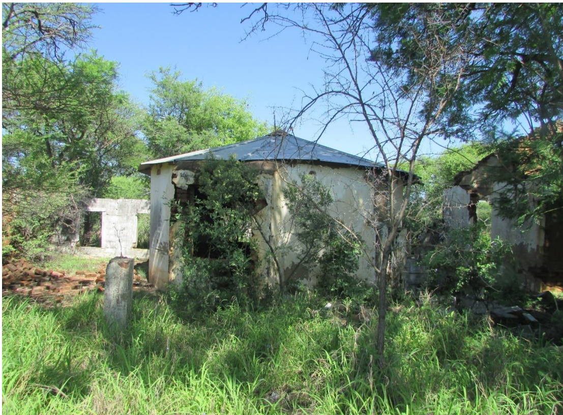
Figure 20: A rondavel structure that formed part of the main homestead.
