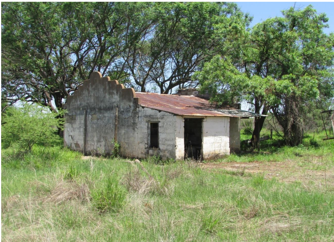
Figure 36: One of the outbuildings on Site 7. This is probably a shed/storeroom. Note the Cape Dutch style gable.
