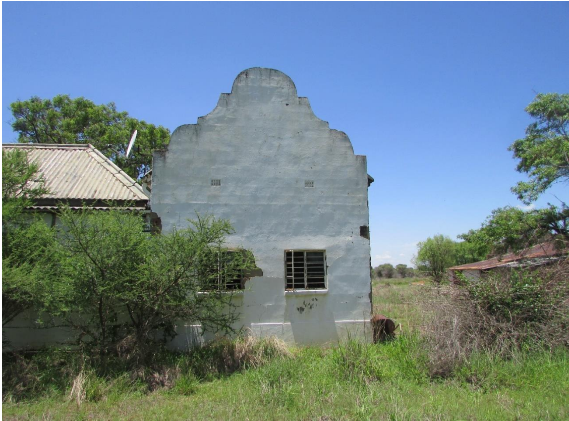
Figure 39: A later addition to the main house. The gable style is Cape Dutch.
