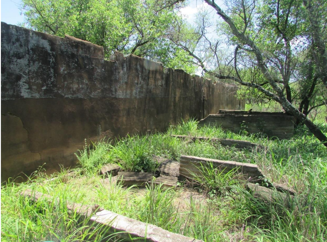
Figure 32: Closer view of a section of the structure in Figure 31.
