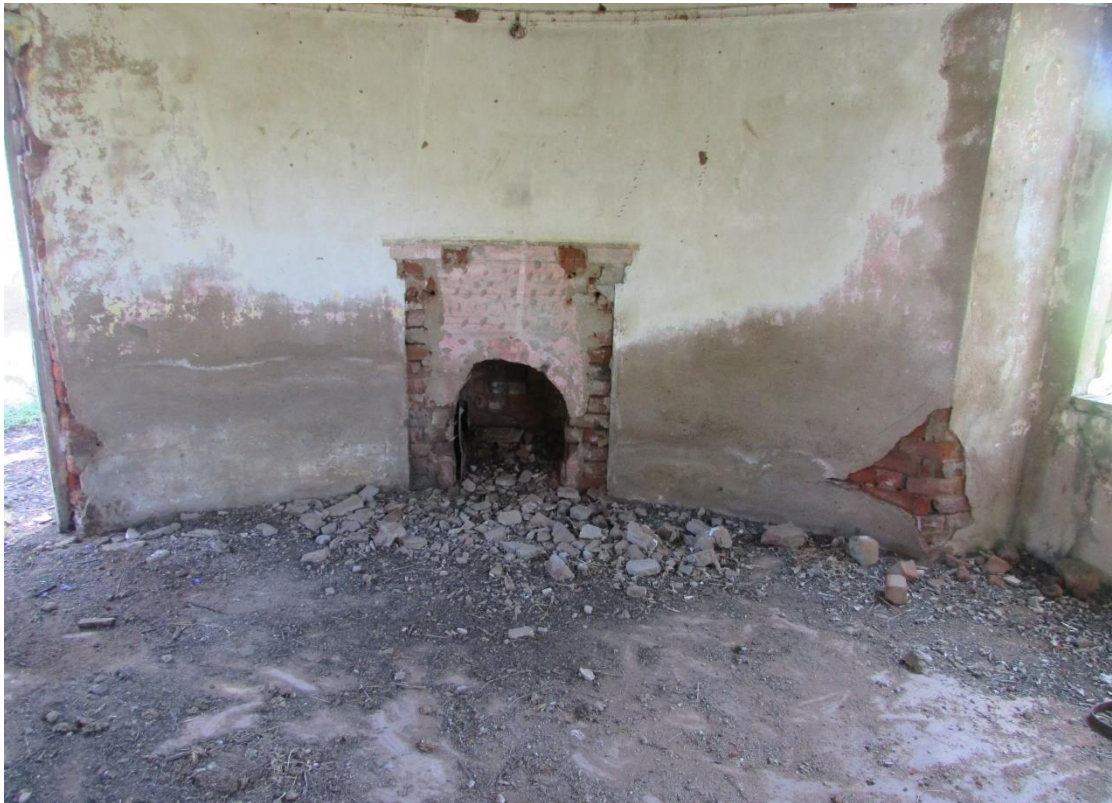
Figure 22: Remnants of the old fireplace/hearth in the main homestead.
