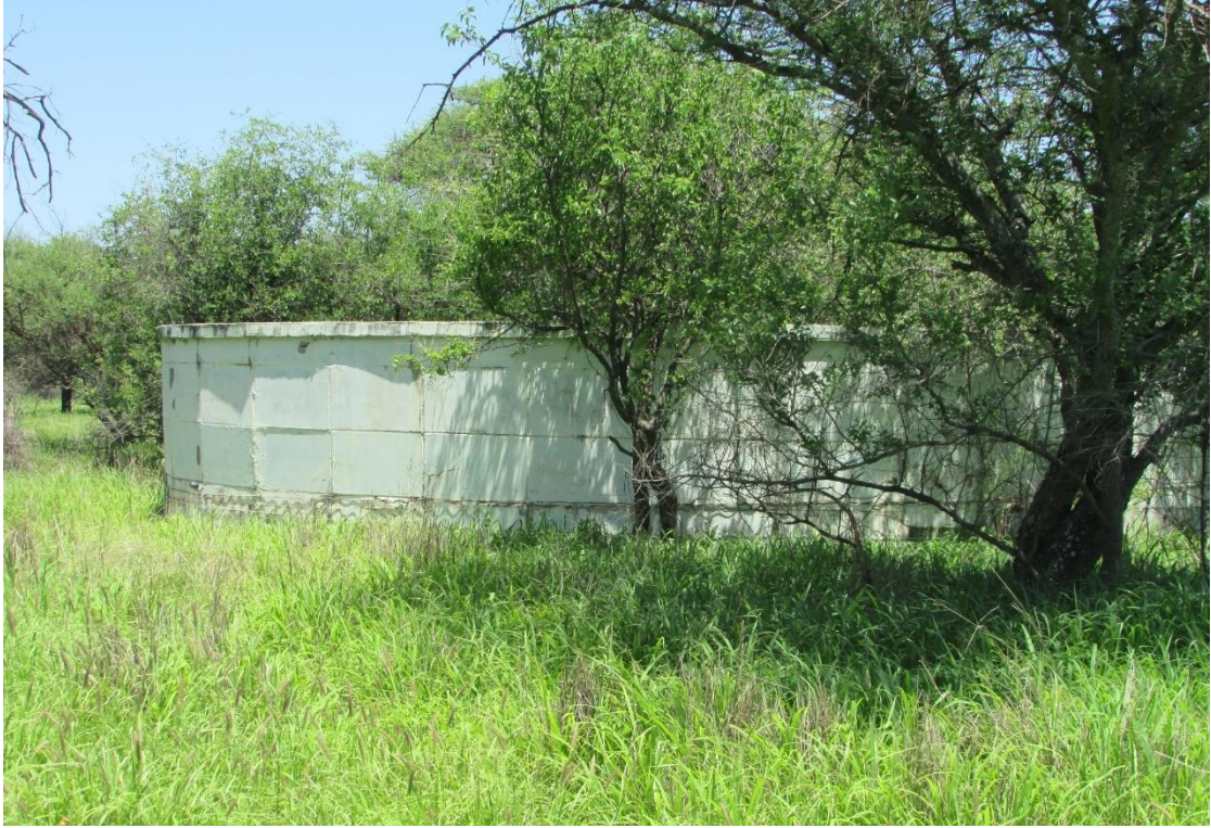
Figure 30: Large steel/corrugated iron dam on the site.
