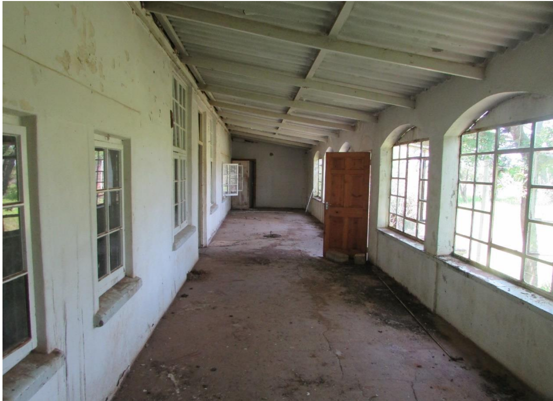
Figure 41: A view inside the house of the enclosed veranda. Originally this would have been open and typical of the wide verandas of farmhouses of the late 19 th /early 20 th centuries.
