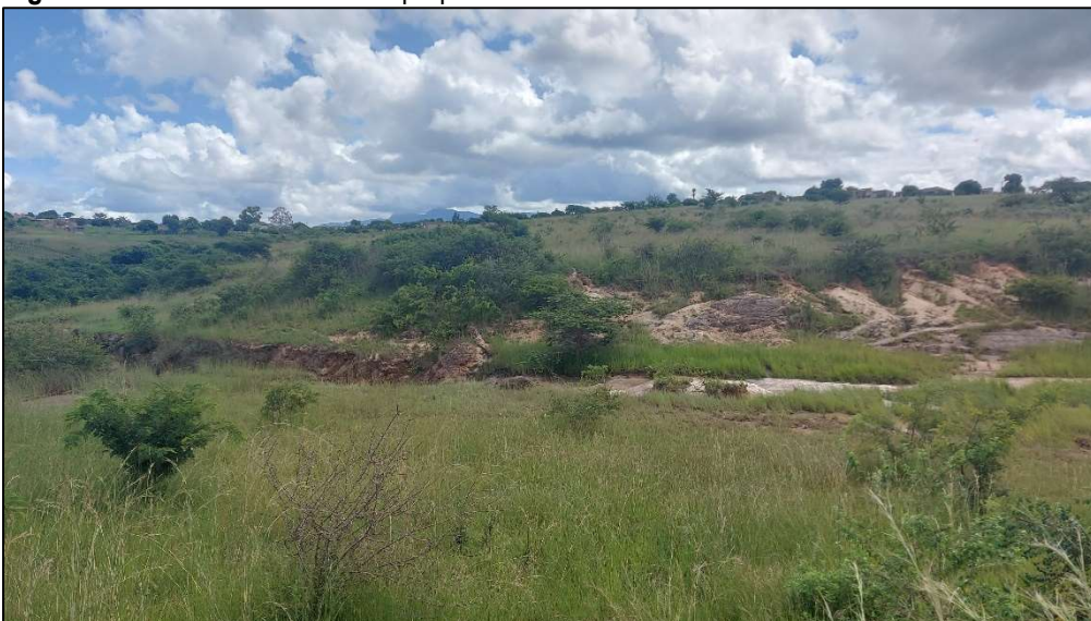
Figure 15: Southern tip of the proposed rehabilitation works area (spillway).
