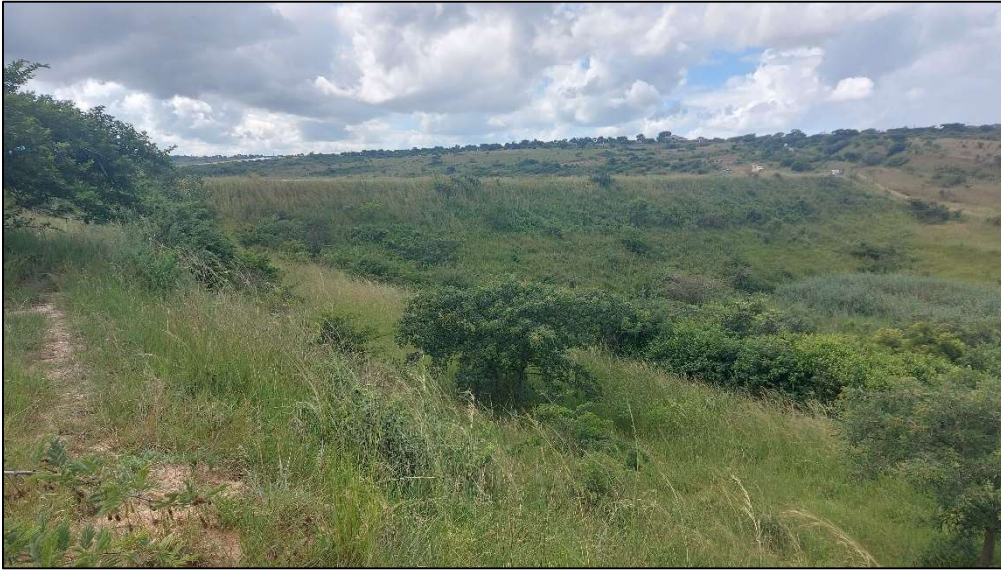
Figure 13: Proposed rehabilitation works area seen from the south (dam embankment).
