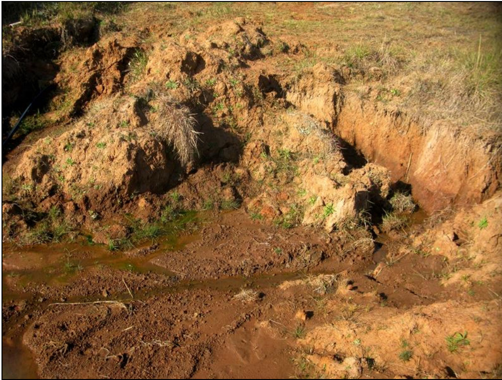
Figure 11. Excavations into thick reddish soils along the eastern edge of the Phase 1 South Area showing small, rounded ferricrete glaebules weathering out of the subsoil profile. Sparse hornfels stone artefacts were recorded within disturbed soils here.
