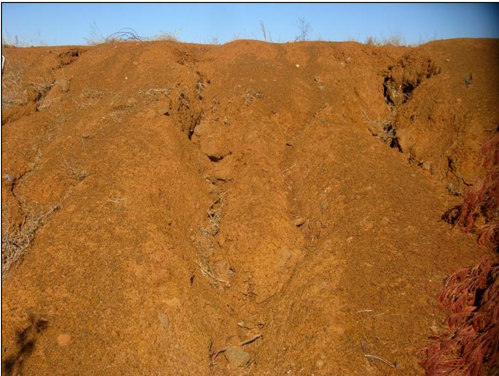
Figure 20. Massive, gullied deposit of sandy to gravelly material and ferricrete glaebules on a steep S-facing scarp just north of the airport runway – probably a result of airport construction activities and not a natural deposit.
