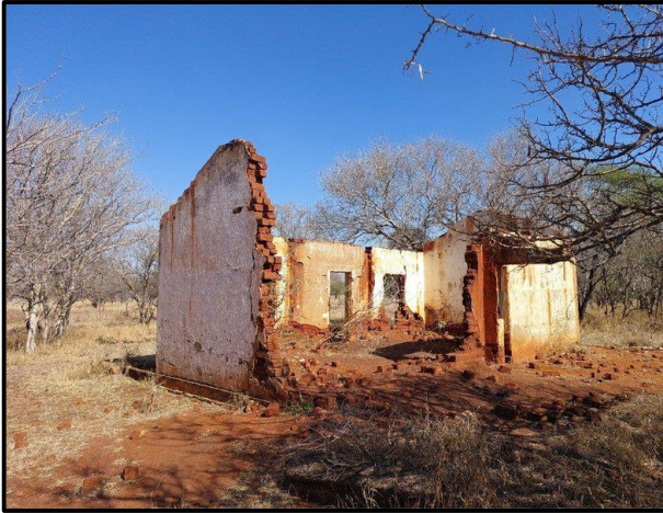
Figure 7.6. Broken down dwelling at DB02.
