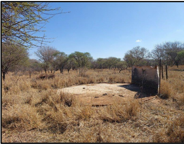
Figure 7.8. Remains of a water reservoir at DB02.
