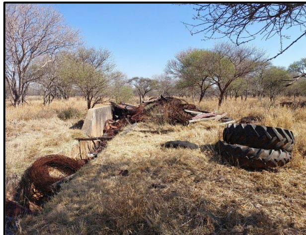
Figure 7.9. Dilapidated dipping bay at DB02.
