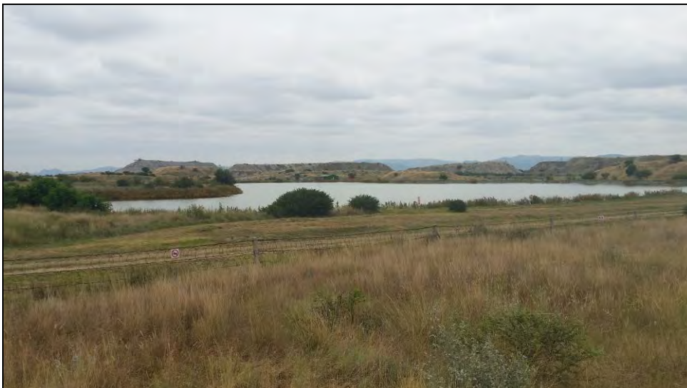
Figure 8: Existing water management systems in the adjacent mining area
