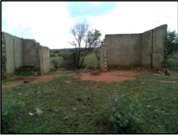
Figure 10: Ruin at Field no 410 viewed from the west
