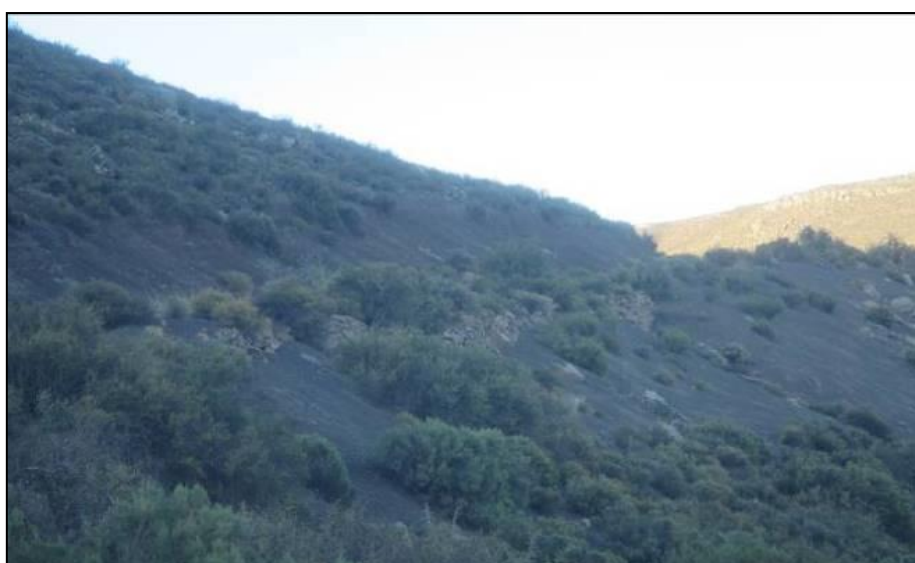
Figure 18: View towards the north showing the road cutting in the slope above the Riet River (waypoint 560).
