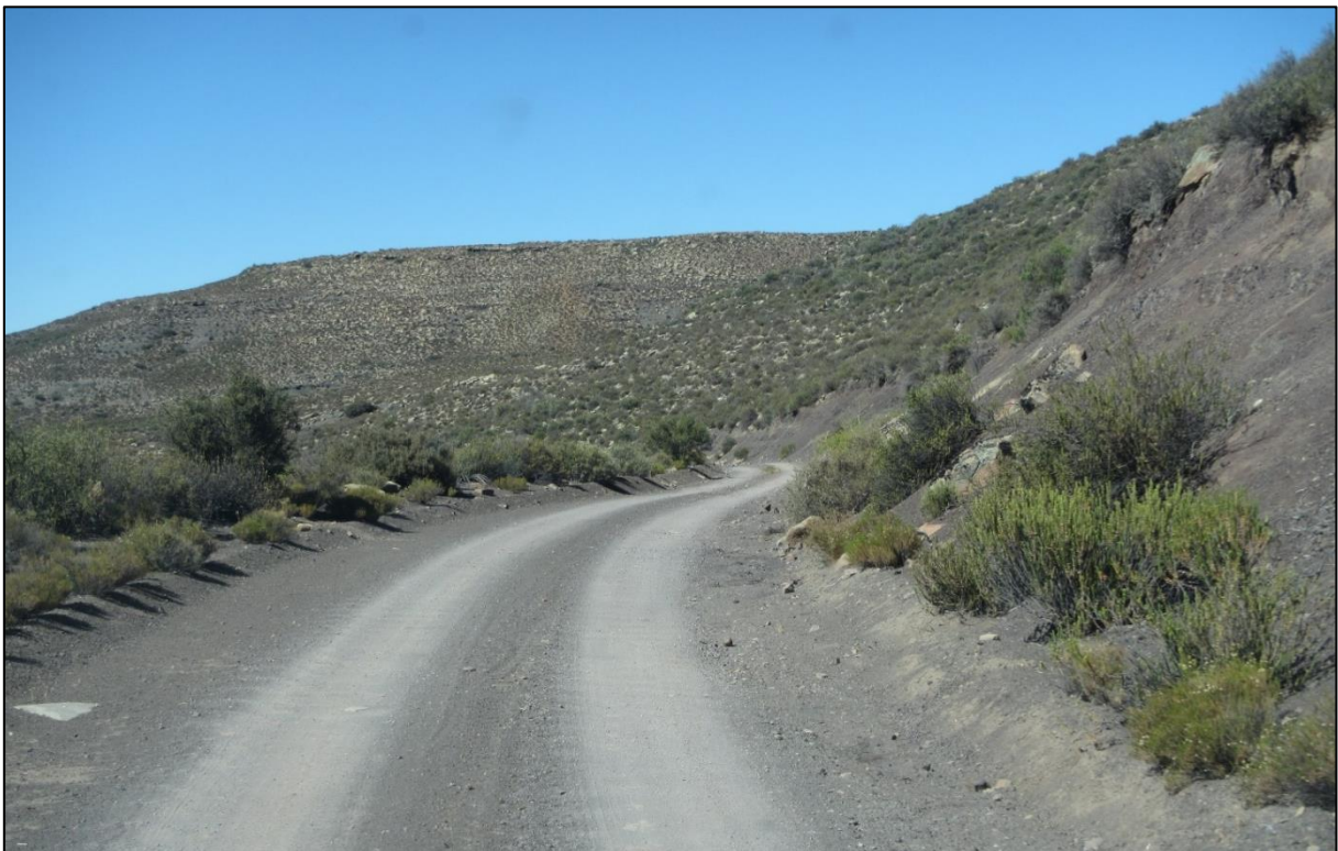
Figure 6: View towards the south in the northern part of the area where the road is cut into the embankment alongside the Riet River.
