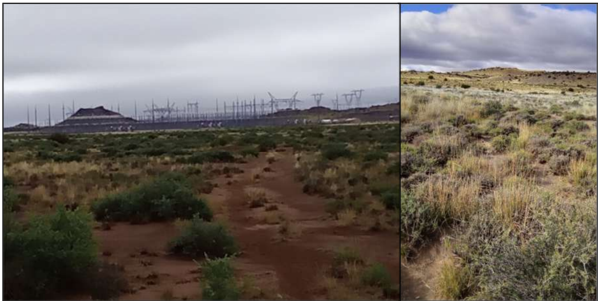
Figure 15: View over Gamma Substation
