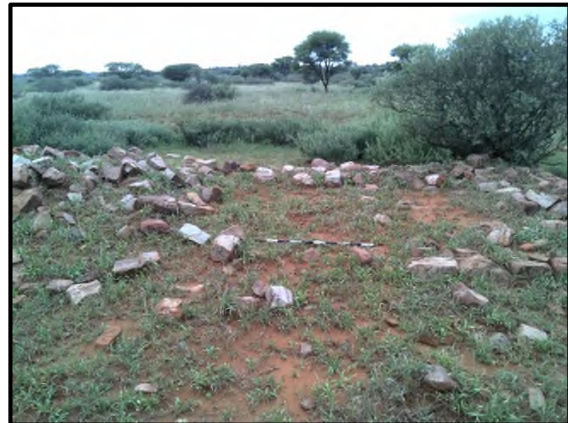
Figure 13: Ephemeral stone foundations at Field No 414
