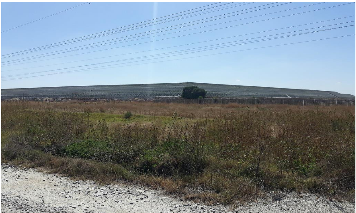
FIGURE 8: MINING INFRASTRUCTURE NORTH OF THE SURVEYED AREA.
