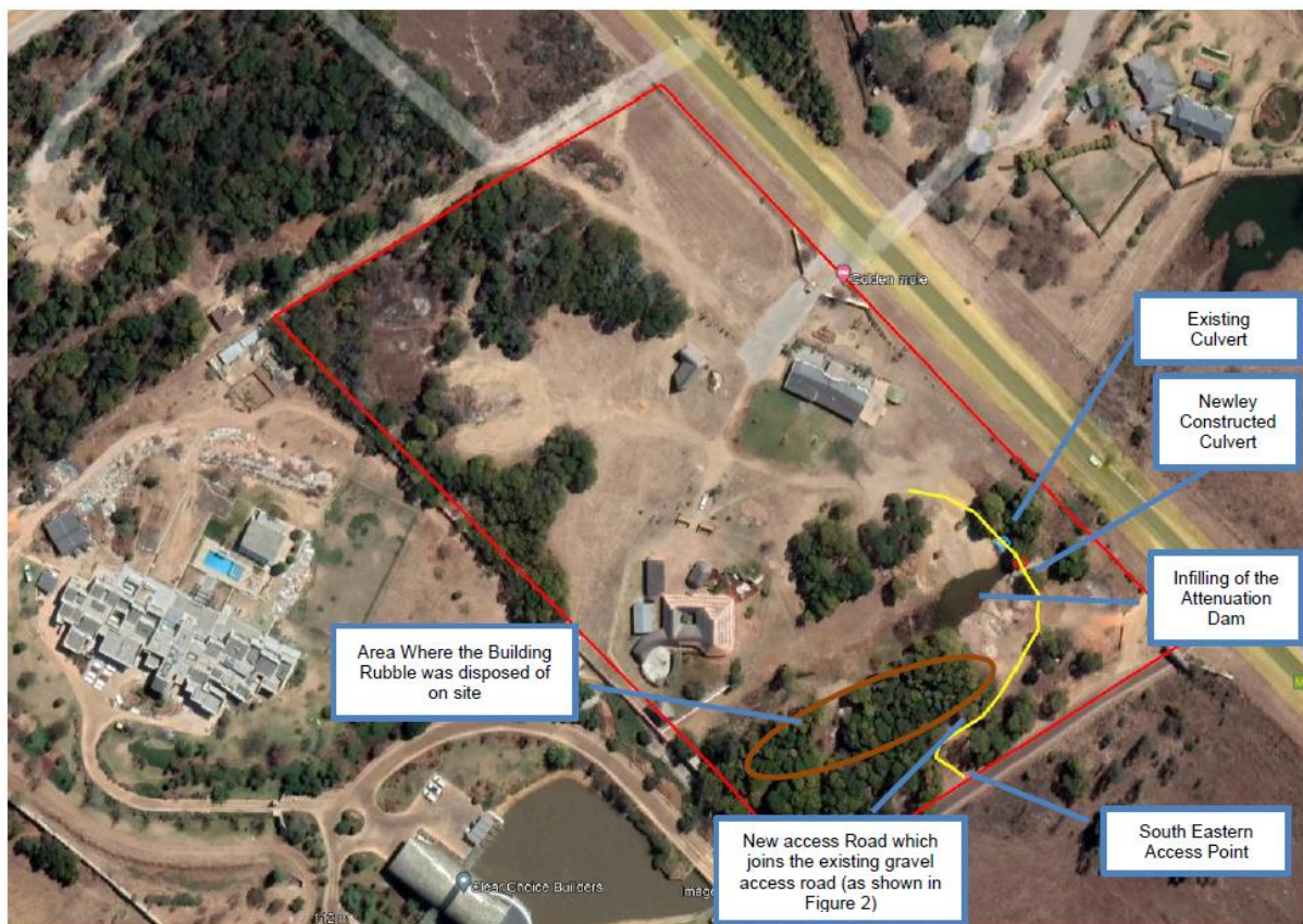
Figure 4: Google Earth Image (2021) showing the construction activities undertaken on site
