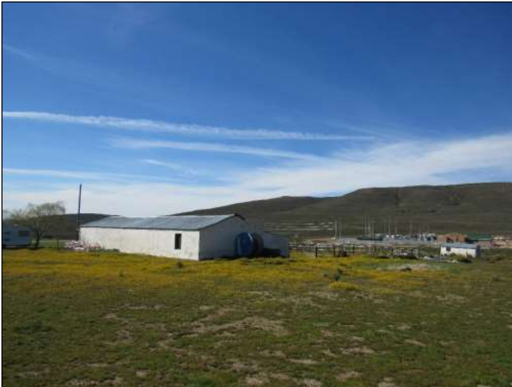
Figure 22: Bon Espirance Substation under construction
