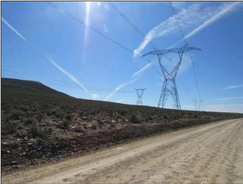
Figure 18: View of high voltage power lines in the study area
