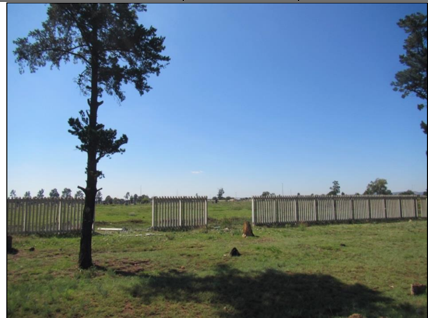
Figure 85 – View of concrete palisade fencing at WTR016
