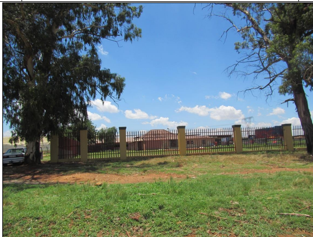
Figure 87 – View of structure and one of the outbuildings
