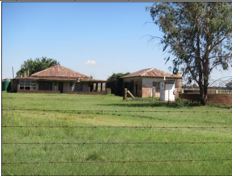
Figure 68 – View of structure and one of the outbuildings
