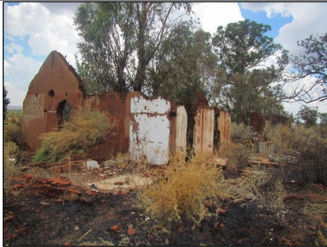
Figure 52 – Alternate view of farmstead
