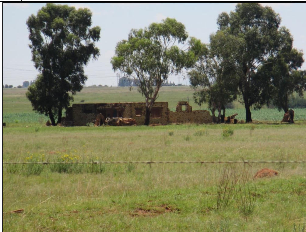
Figure 86 – View of the structural remains at WTR017
