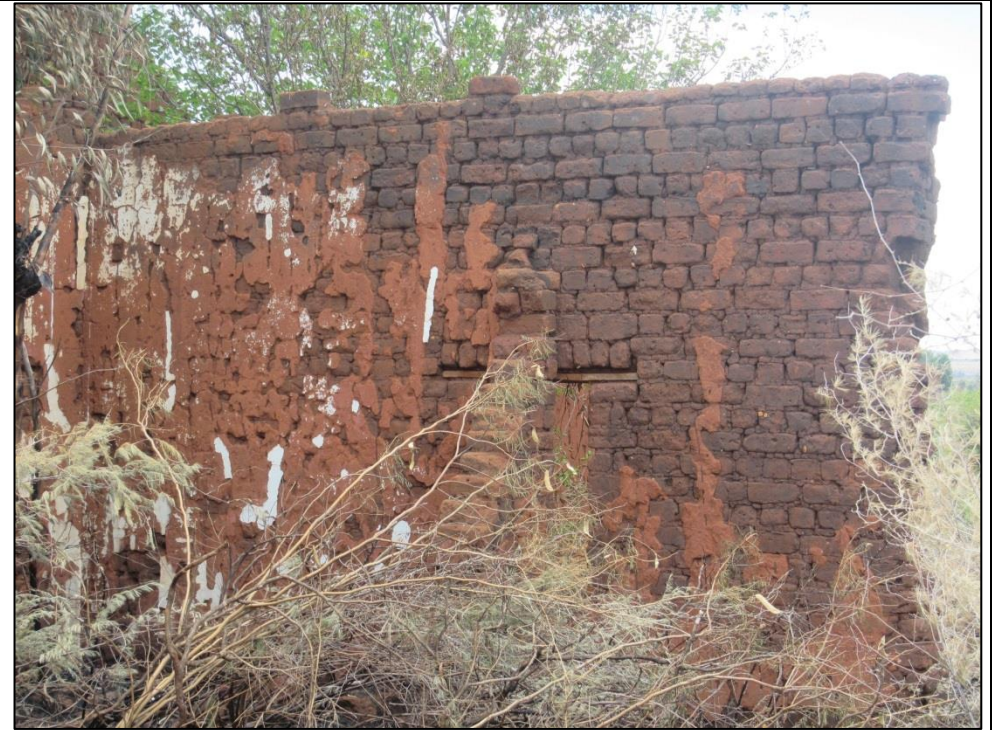
Figure 57 – One can see the 'header-stretcher' bricklaying technique
