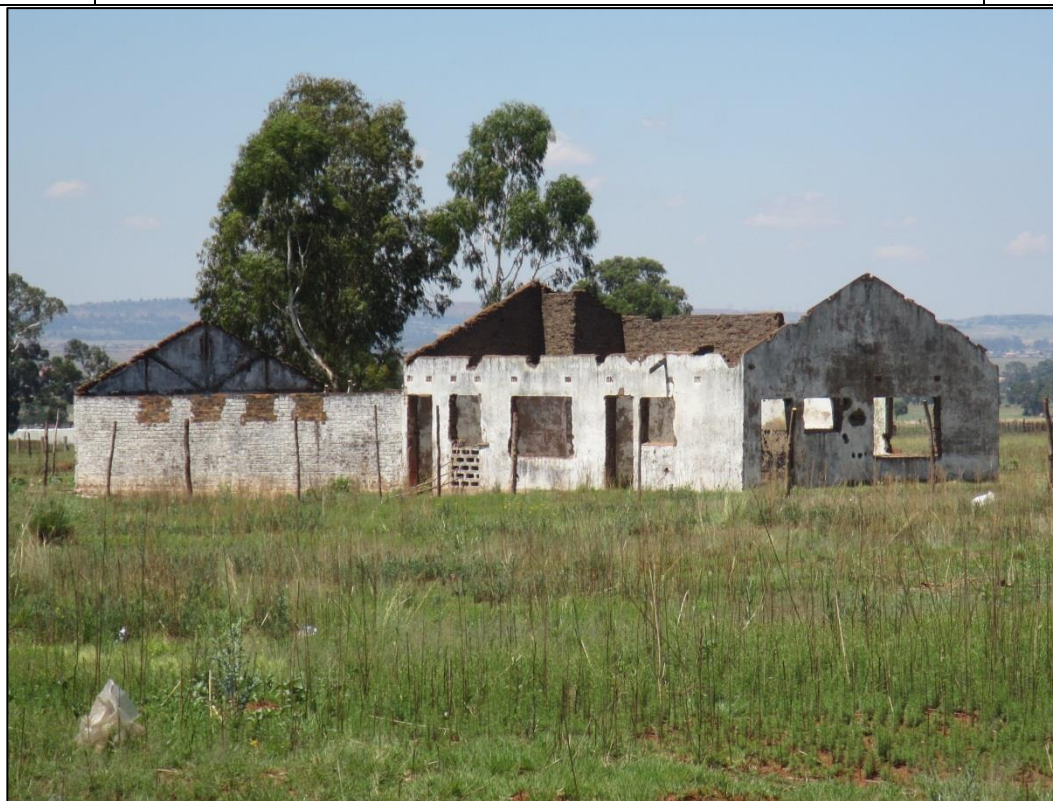
Figure 83 – View of structure and one of the outbuildings
