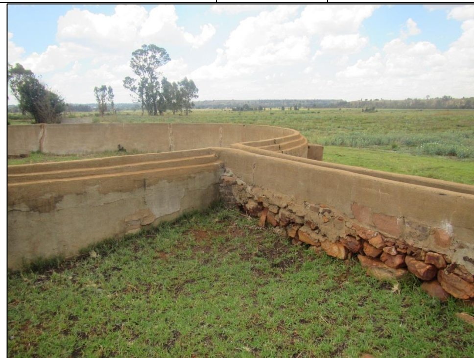
Figure 59 – Circular reservoir and upper portion of spillway
