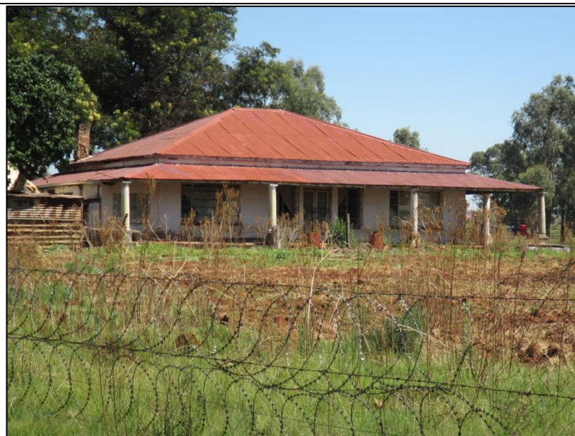
Figure 71 – View of the structure at WTR012
