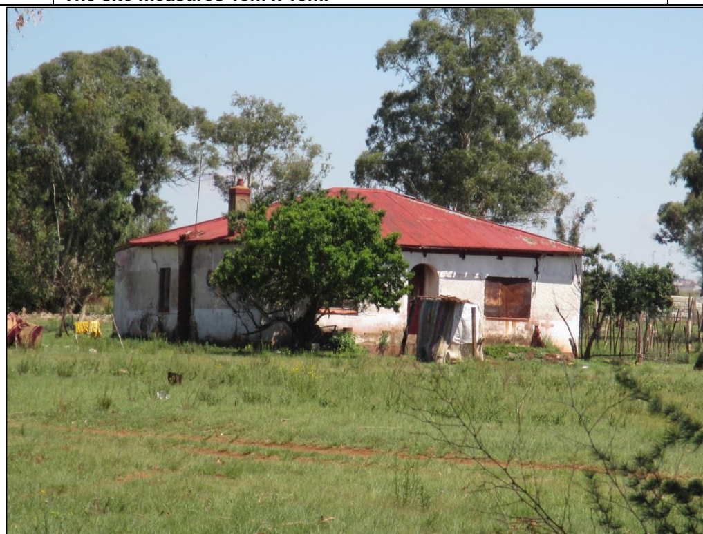
Figure 70 – View of structure at WTR011
