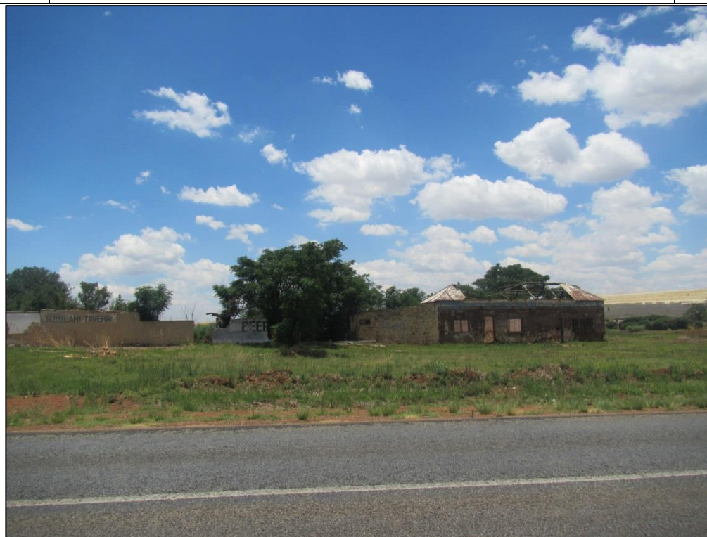
Figure 88 – View of structure and one of the outbuildings
