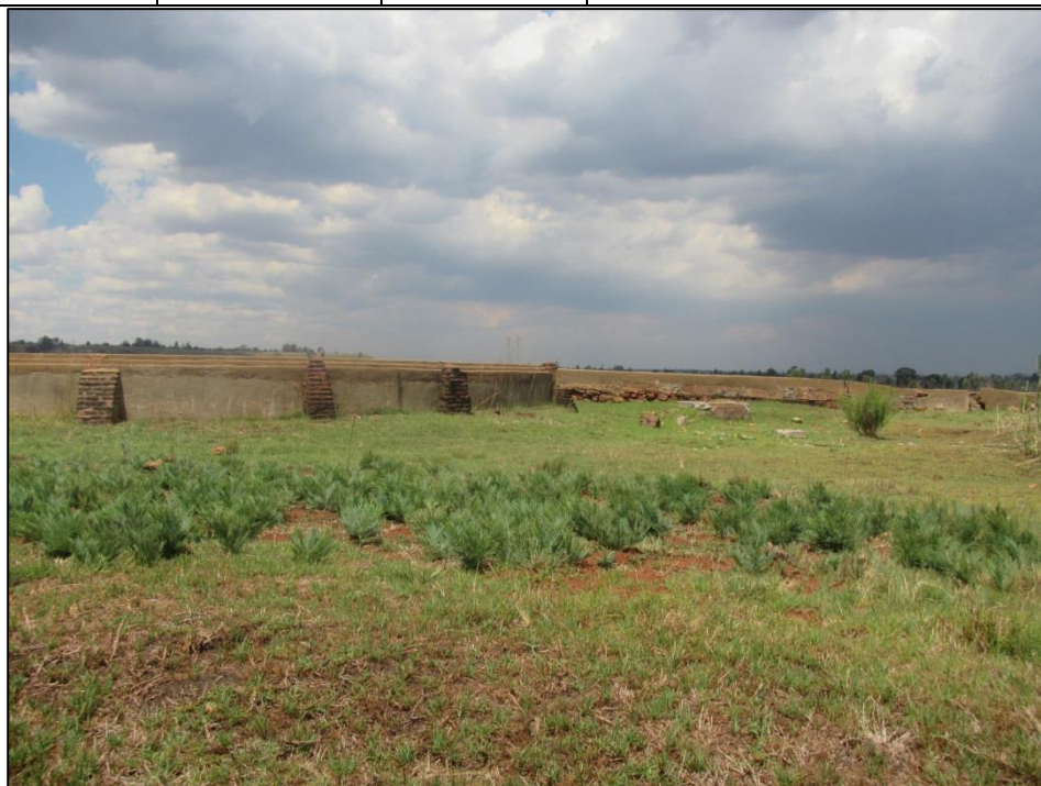
Figure 58 – Overall view of reservoirs and spillway at WTR007
