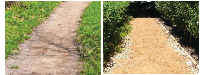
Informal compacted laterite / insitu soil pathways
