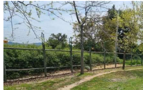
Estate perimeter fence: visually permeable steel mesh fencing type with timber posts and additional security above.
