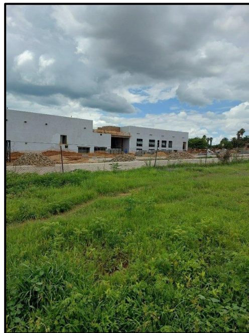
Figure 7.4. Active construction site on the northern boundary of the project area.
