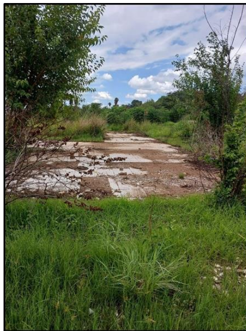
Figure 7.8. Modern foundations of demolished ruins scattered across the eastern edge of the project area. - Image shows the foundation marked DP001
