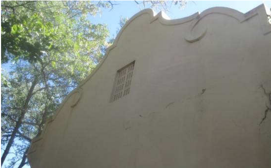
Figure 12. The south western Cape Dutch Gable of the 1920's period farmhouse.
