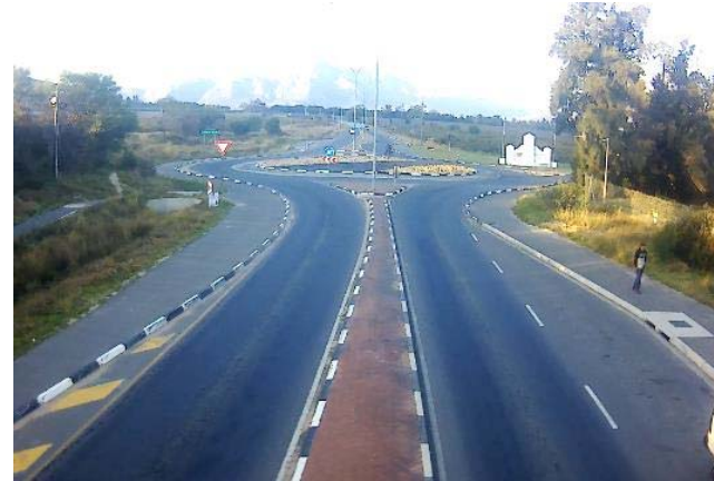
Photo 10: Southbound View along R301 (MR201) approaching Kliprug Minor Road Roundabout
