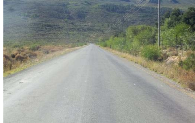
Photo 6: Eastbound view along Schuurmansfontein Road from Access 1 location
