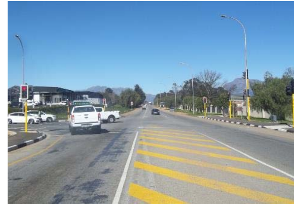
Photo 2: Southbound View along R301 approaching Lustigan Road
