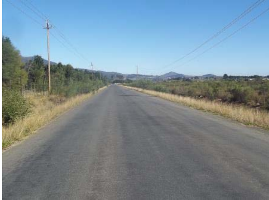
Photo 5: Westbound view along Schuurmansfontein Road from Access 2 location
