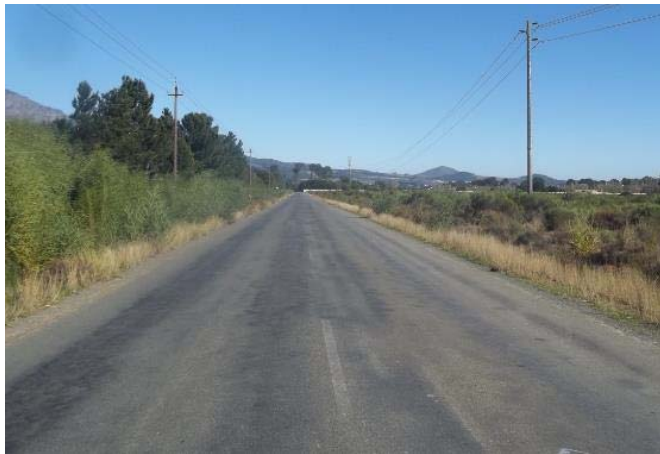
Photo 7: Westbound view along Schuurmansfontein Road from Access 1 location
