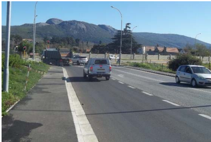
Photo 3: Westbound view along Lustigan Road approaching the R301 (MR201)
