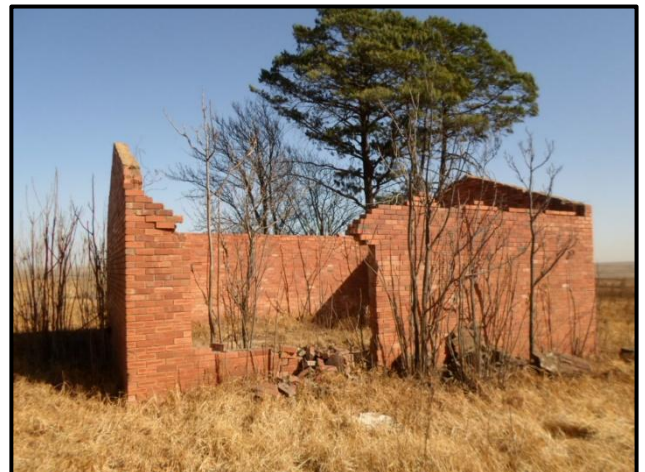
Figure 15. Red brick structure viewed from the west
