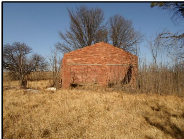
Figure 14. Red brick structure viewed from the north
