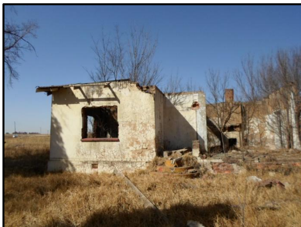
Figure 16. Main dwelling viewed from the north east
