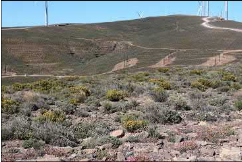
Figure 8: New wind farm infrastructure on Ekkraal 199, some 2 km west of the new Eskom substation on Bon Espirance 93, showing the substantial area of surface disturbance associated with even small-scale overhead powerlines (middle ground). Sectors of wind turbine access road also require the excavation of major new road cuttings into Abrahamskraal Formation bedrocks.
