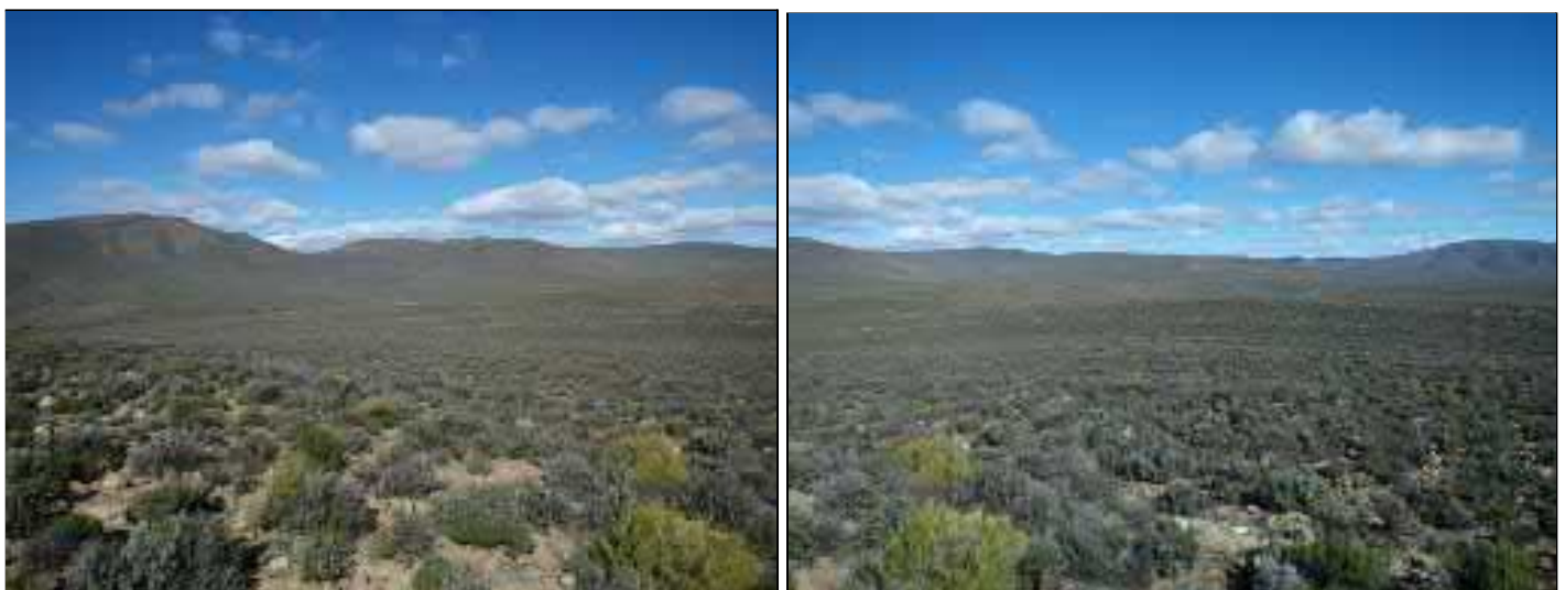
Figure 4.4: Contextual Images taken from the substation location in the west with existing turbines visible on the ridgeline
