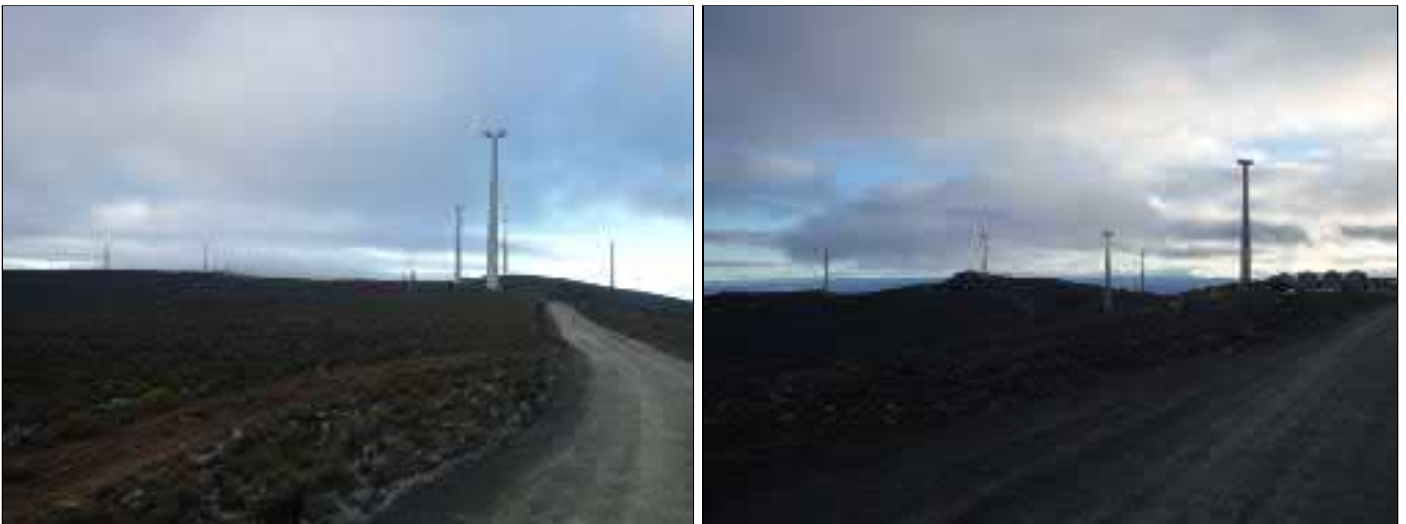
Figure 4.6: Contextual Images taken from the alignment running north-west to south-east indicating turbines under construction
