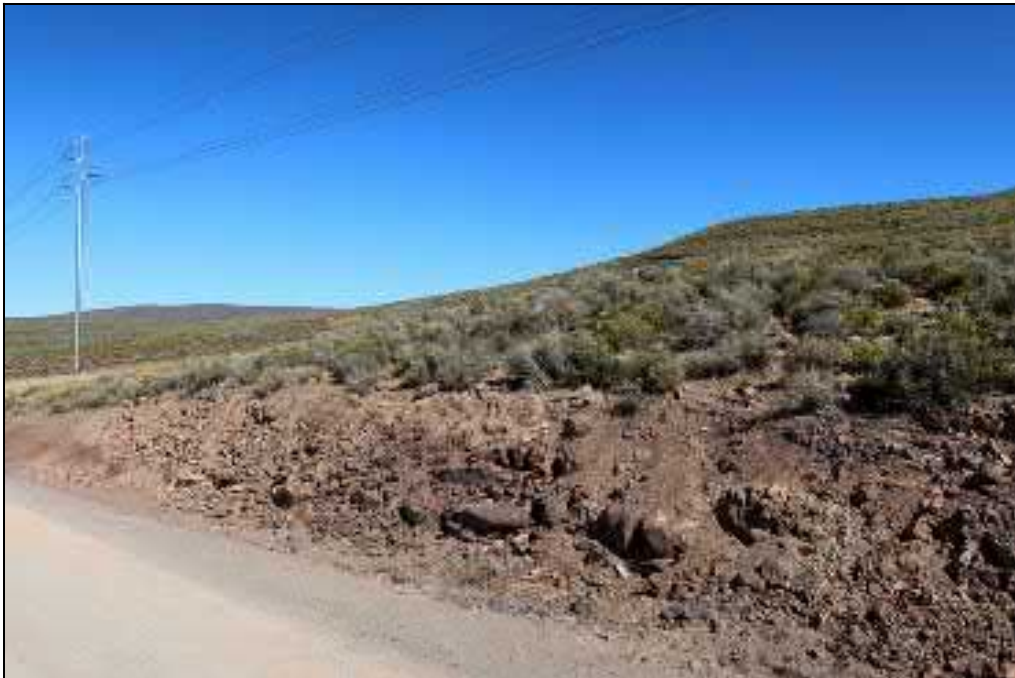
Figure 9: New road cuttings into maroon mudrocks along the access road to the Eskom substation on Bon Espirance 73. In practice, the recognition, sampling and recording of fossils within freshly-exposed bedrock sections is often highly problematic due to soils / dust cover and fragmentation during excavation.
