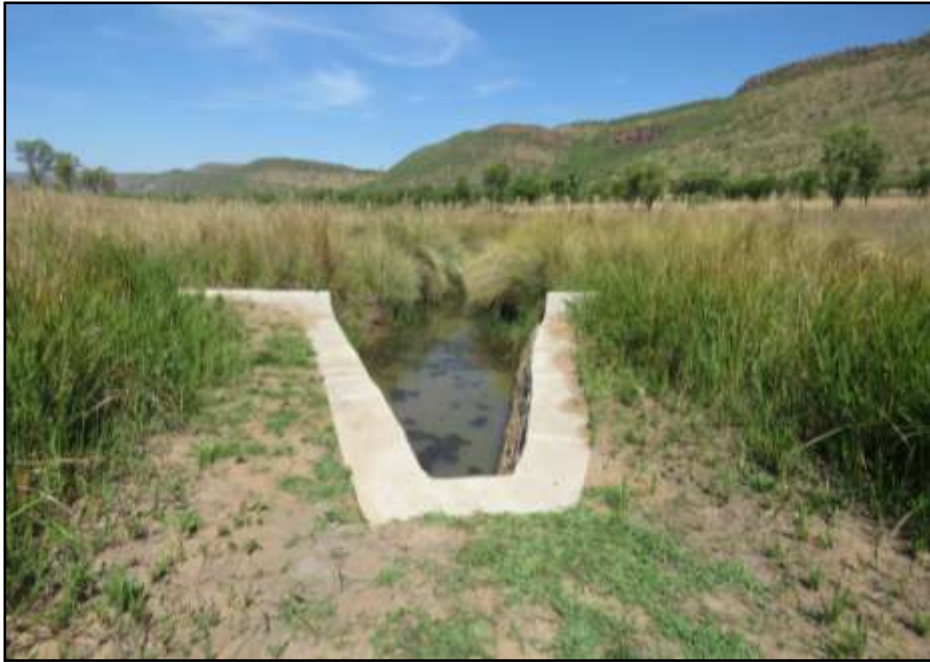
Fig. 1. An example of a typical hard engineering intervention known as a stone masonry weir which may be used at Hondekraal.
