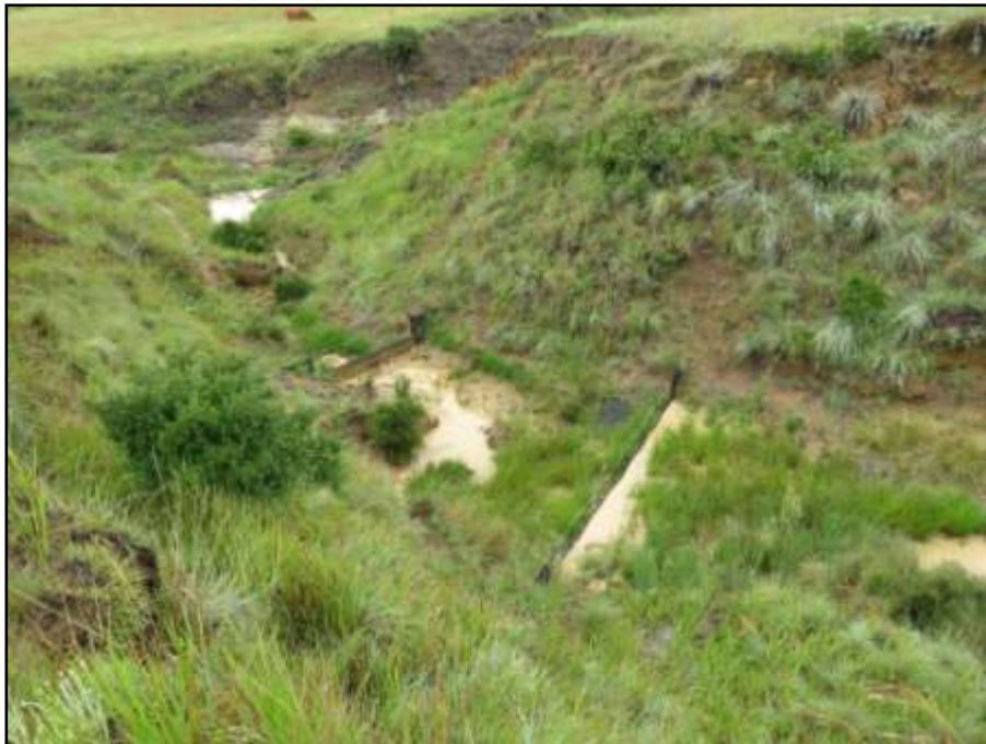
Fig.4. Silt fences after it has been implemented in an erosion donga resulted in halting the erosion and re-established plant growth.
