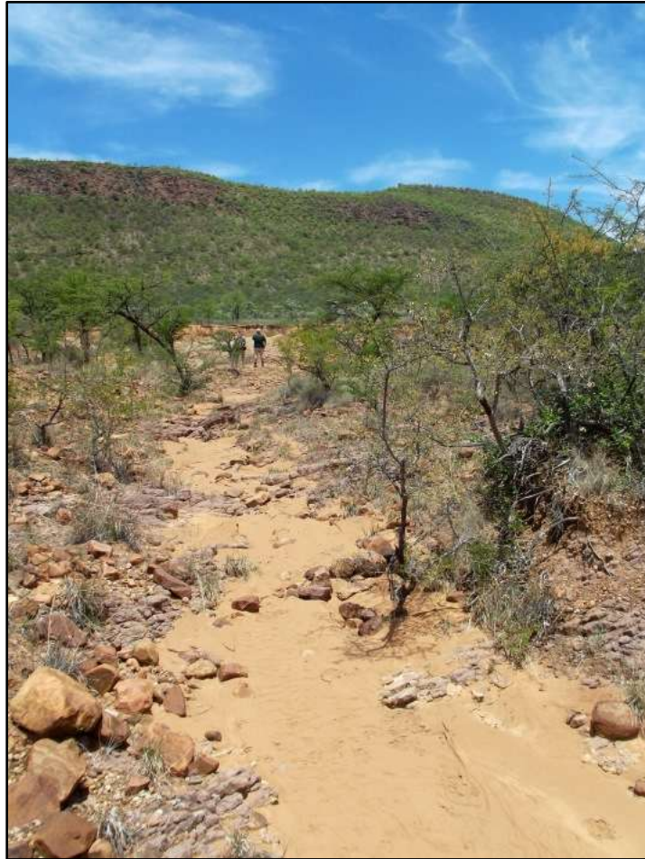
Fig. 17. Site D. Approximately 100m north of site D where the silting is obvious. This is potentially a place where a “hard intervention” structure can be placed.
