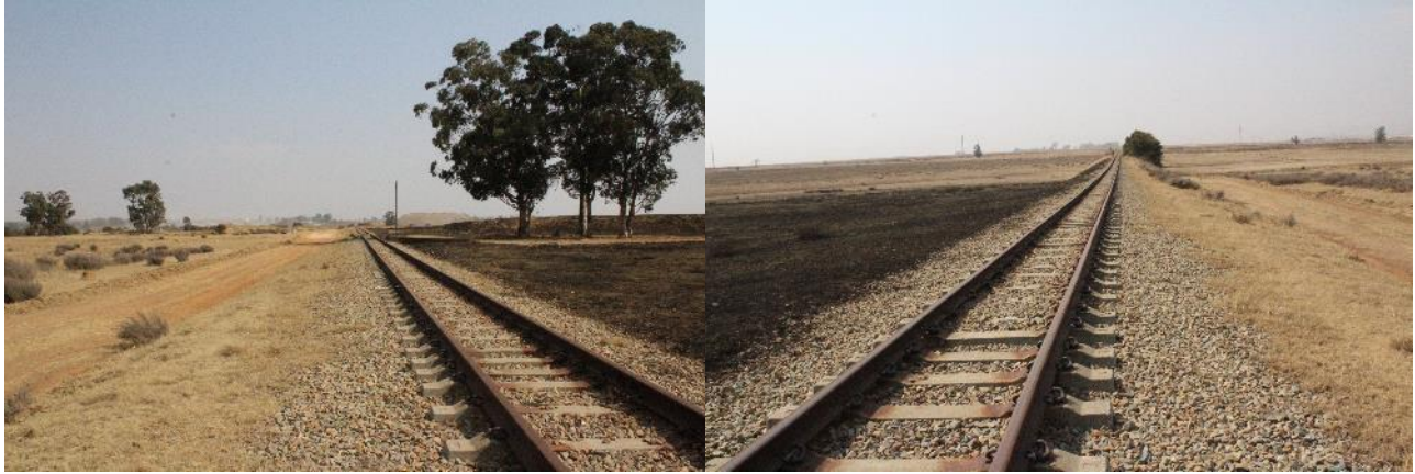
Figure 6: Train tracks located near the southern section of the pipeline
