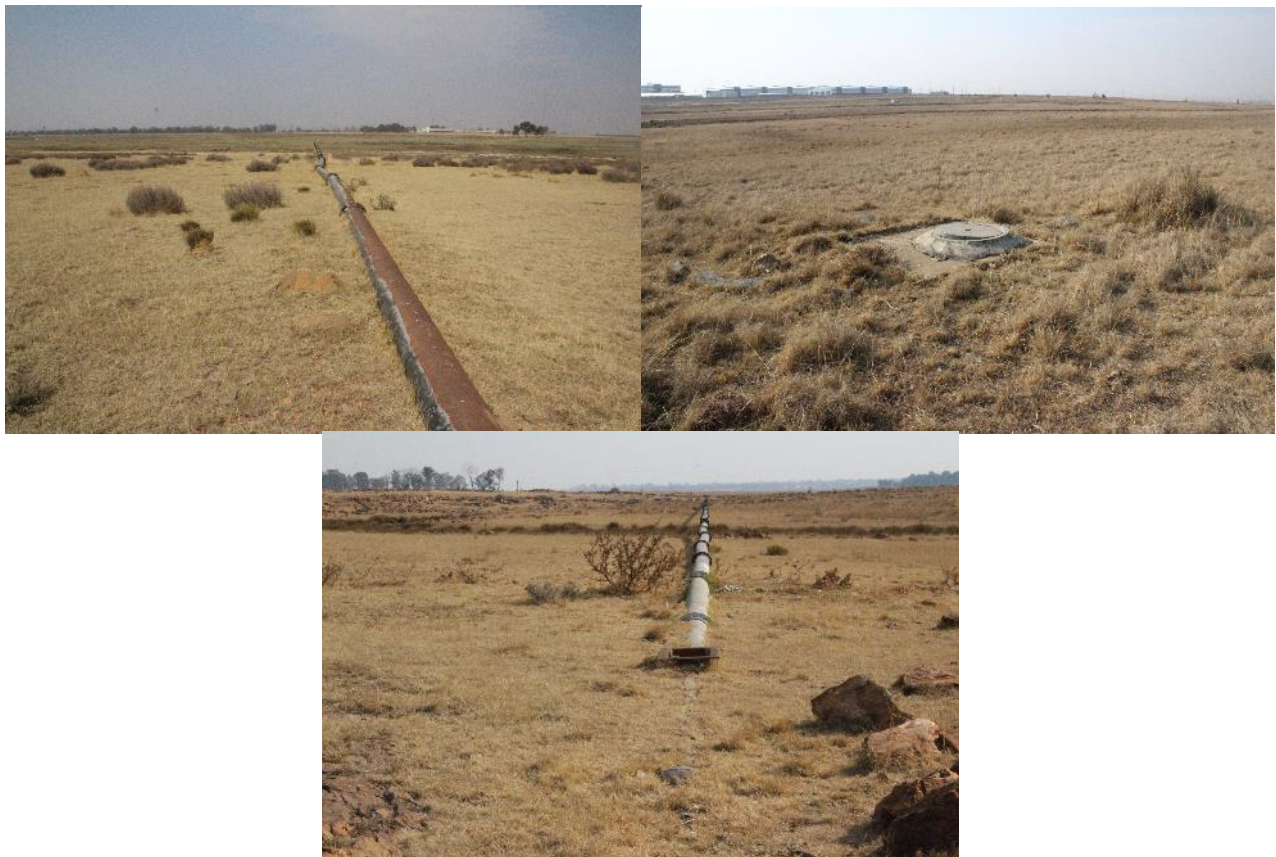
Figure 5: Sewer pipes running through the project area
