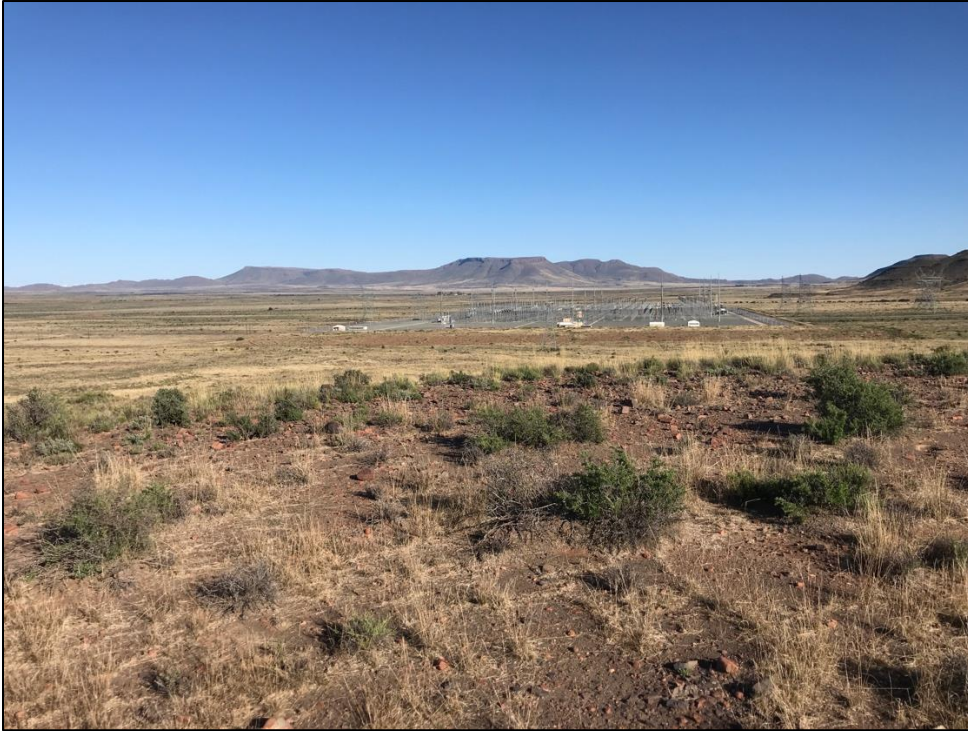
Figure 21 - View towards the existing Gamma Substation.
