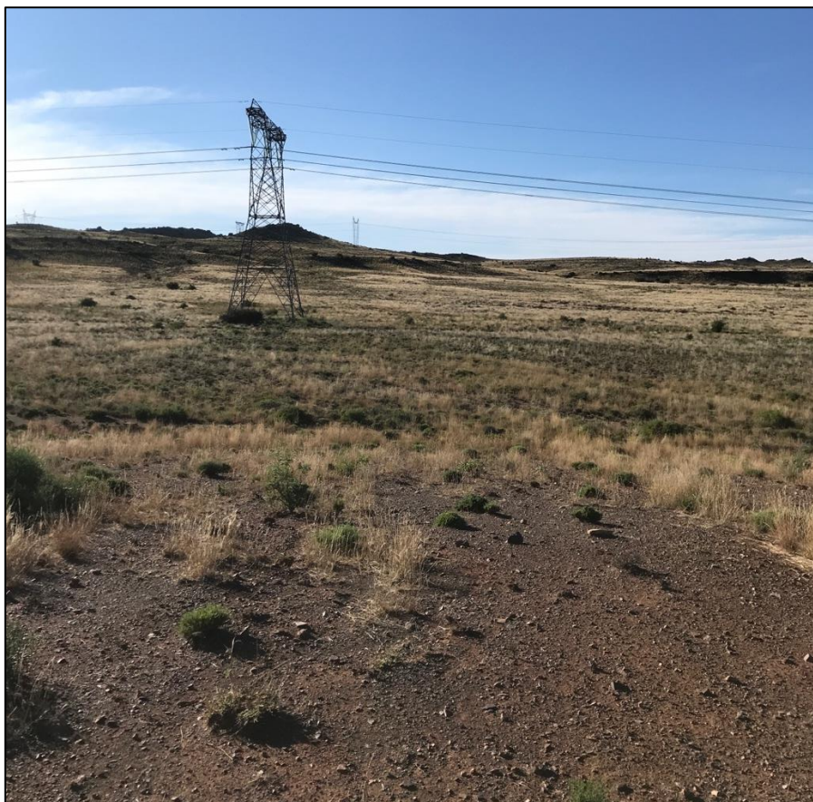
Figure 19 - View of the existing powerline in the region.
