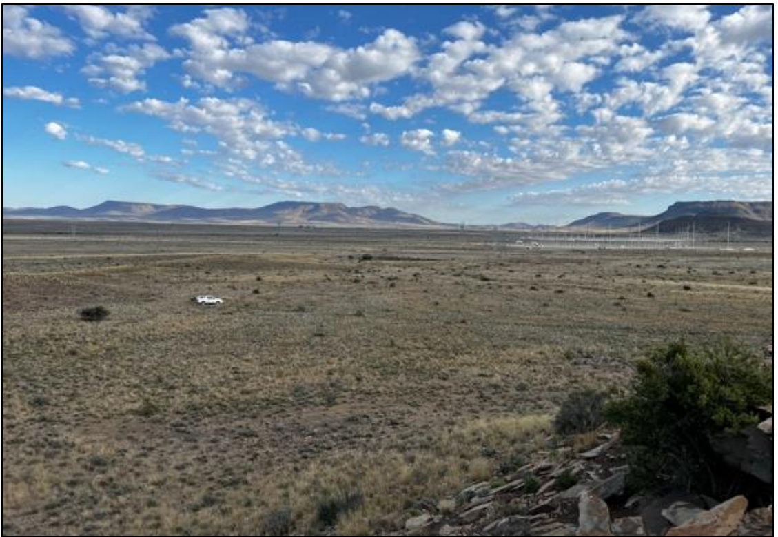
Figure 9 - View towards the existing Gamma Substation.
