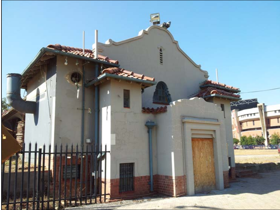
Figure 2: Western facade of the Clubhouse, 2012
