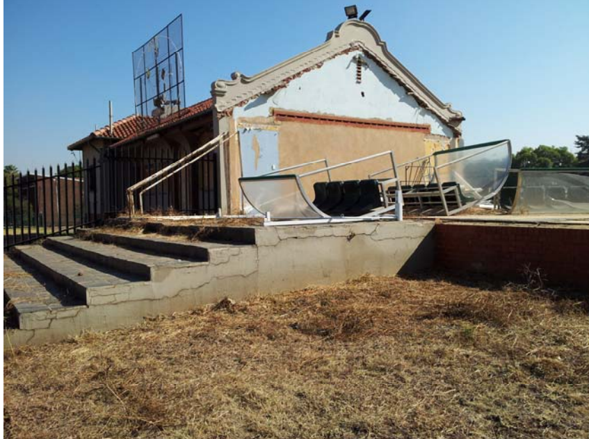
Figure 8: Eastern facade indicating the remains of the eastern addition
