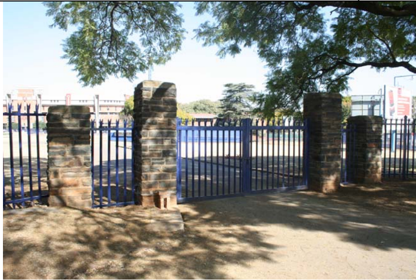
Figure 12: Stone Entrance Gate to the Sports Ground
