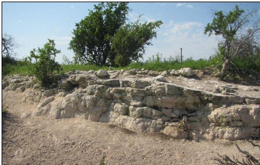
Figure 28: Cutting through calcrete along the east side of the R27 within corridor occupied by all three transmission alternatives.
