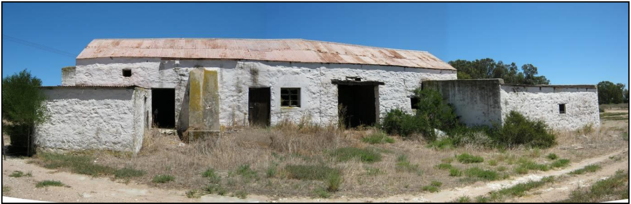
Figure 14: A typical stone-walled, tin-roofed vernacular farm structure on the farm Uyekraal 189 (Source: Orton 2011:figure 14).
