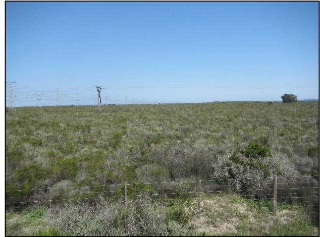
Figure 10: View towards the south from the R45 with the Aurora Substation behind the viewer.
