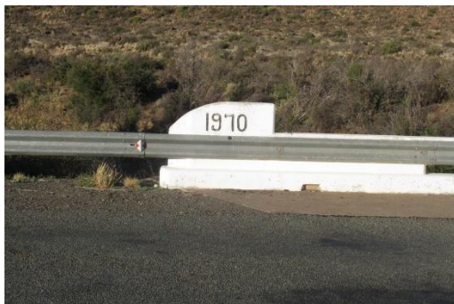
Pylon, indicating the bridge date
