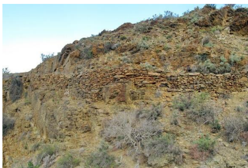
Terrace walling forming walkway
