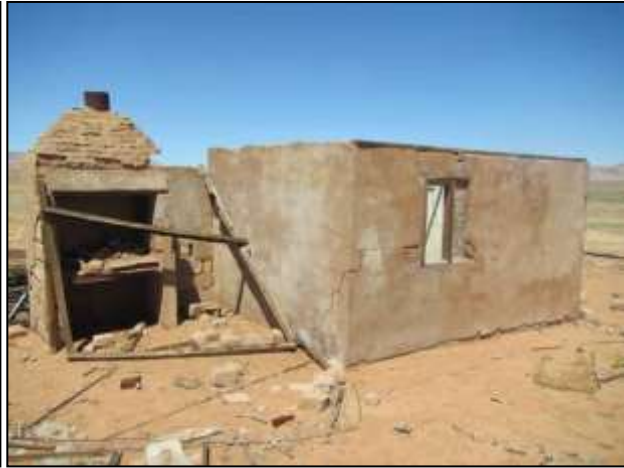
Figure 29: The cottage with external hearth at waypoint 008.
