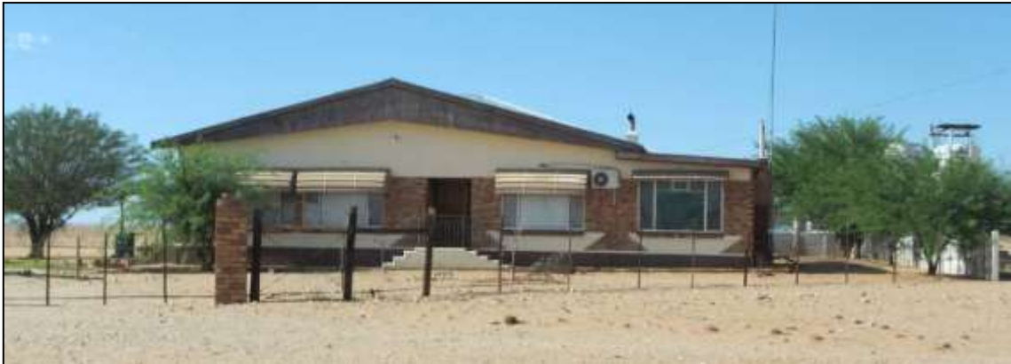
Figure 25: House forming part of the Ou Taaibosmond farm complex.
