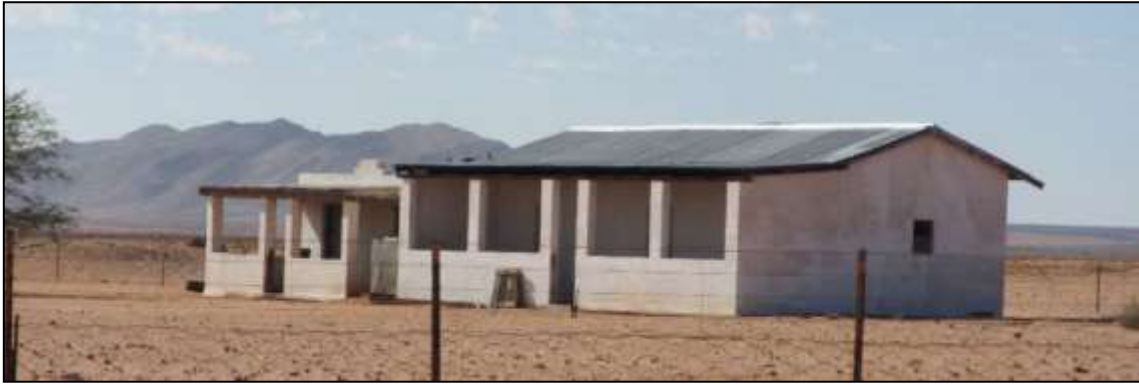
Figure 23: House forming part of the Ou Taaibosmond farm complex.
