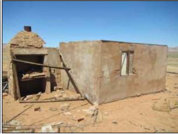
Figure 29: The cottage with external hearth at waypoint 008.
