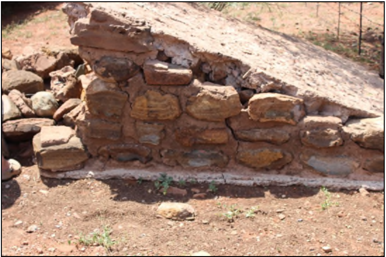
Figure 8. Several stromatolites were used to build a ramp. These stromatolites were most probably collected in the development area. See Figure 5 for the location of the ramp within the Remaining Extent of the farm Woodhouse 729.
