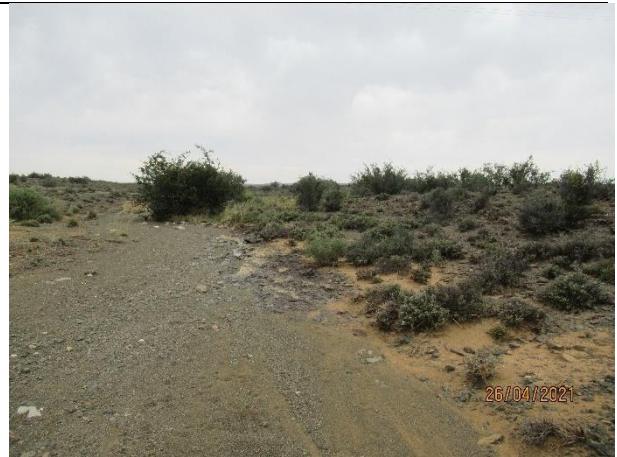
Major culvert 1/3/1mx2.3m
