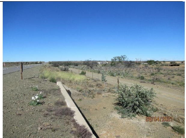
Major culvert 1/3.2mx2.4m
