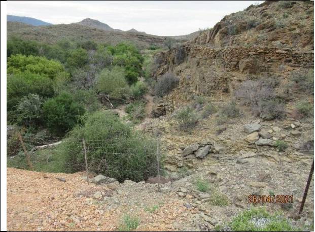
River bridge 3/8.2mx3.7m
