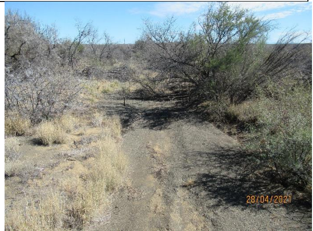
Major culvert 3/3.4mx1.9m
