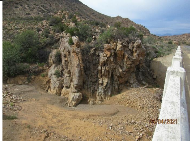
River bridge 5/11.1mx3.4m
