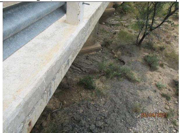
Major culvert 2/3.8mx3.9m
