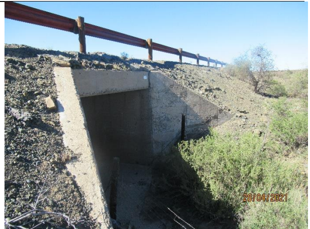
River bridge 3/3.5mx3.7m
