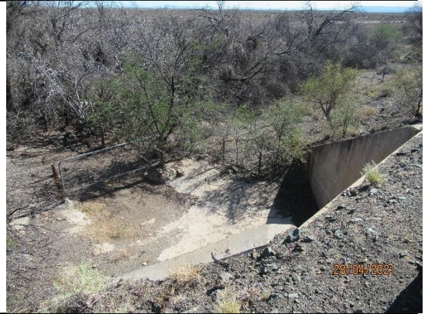
Major culvert 2/2.7mx2.1m
