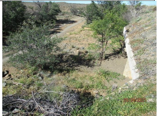
Major culvert 4/3.1mx1.2m
