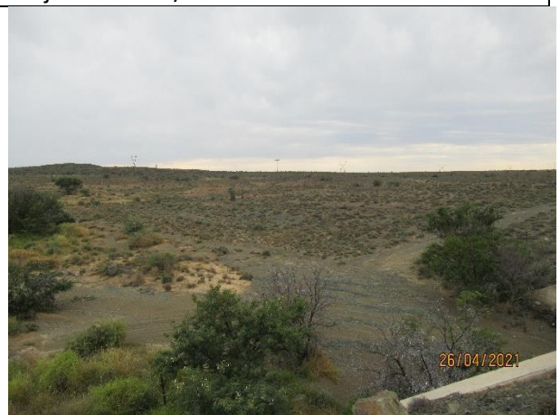
Major culvert 1/3.1mx2.1m
