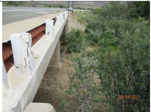
Major culvert 2/1.8mx1.8m
