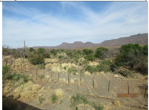
Major culvert 305ø
