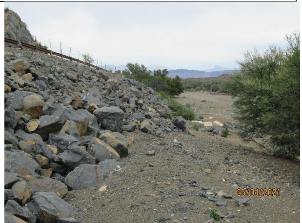
Major culvert 2/1.8mx1.8m
