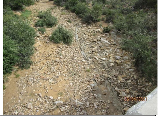
River bridge 3/7.6mx4.9m
