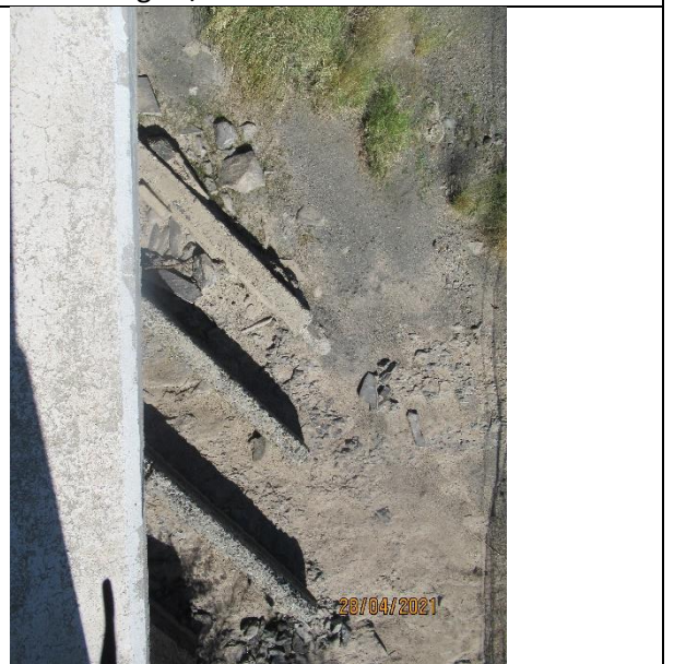
Major culvert 2/2.9mx1.8m
