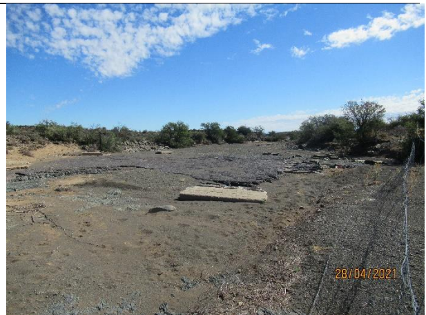
River bridge 3/76mx3.0m
