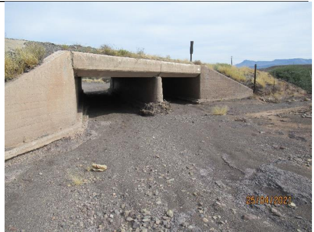
River bridge 6/5mx1.6m
