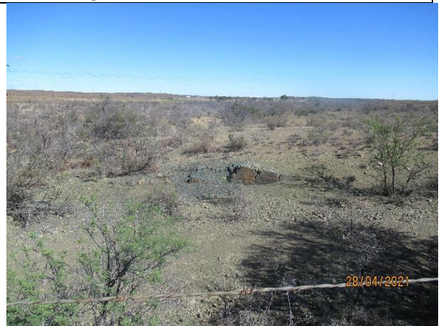
Major culvert 1/2.5mx1.8m
