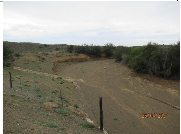
River bridge 1/6.8mx6.1m
