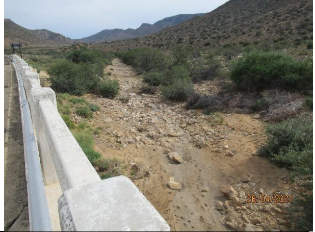
Major culvert 1/3.7mx3.4m
