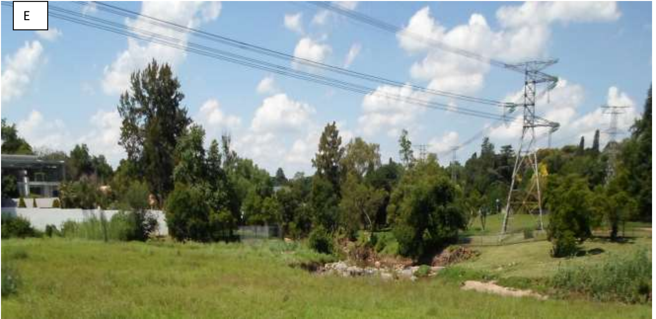
Plate 7: Photo E. showing project area is within electricity distribution servitude
