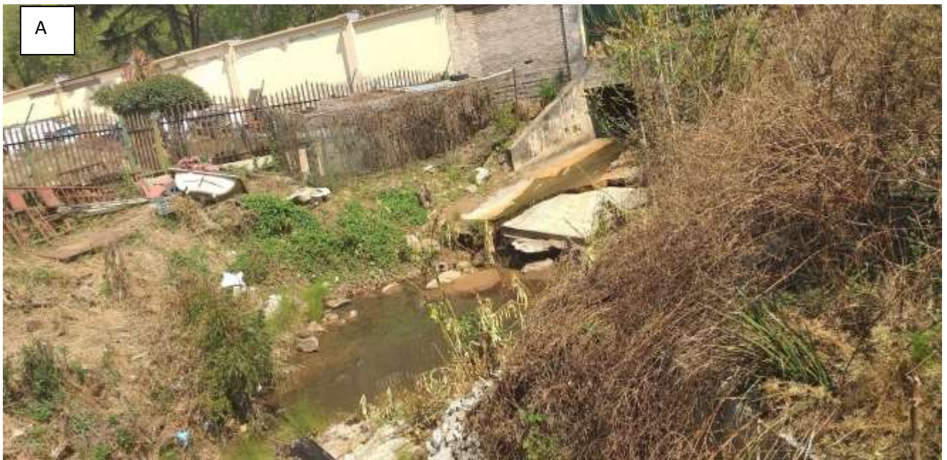
Plate 1: Plate 2: Photo A. View of canal to be rehabilitated
