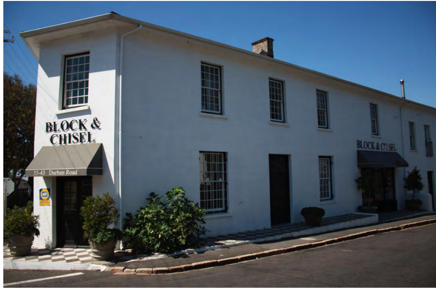
Figure 44: Wynberg Village: The Use of 'Wall-like' Architecture
