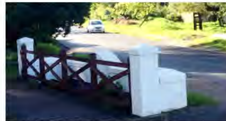
Fig. 34 Culvert crossing and footbridge (Briel, 2015)
