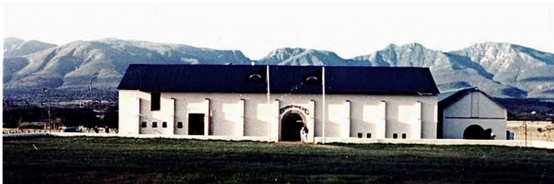
Fig. 112 Market building example Martin Kruger Architects - Birkenhead Brewery.
