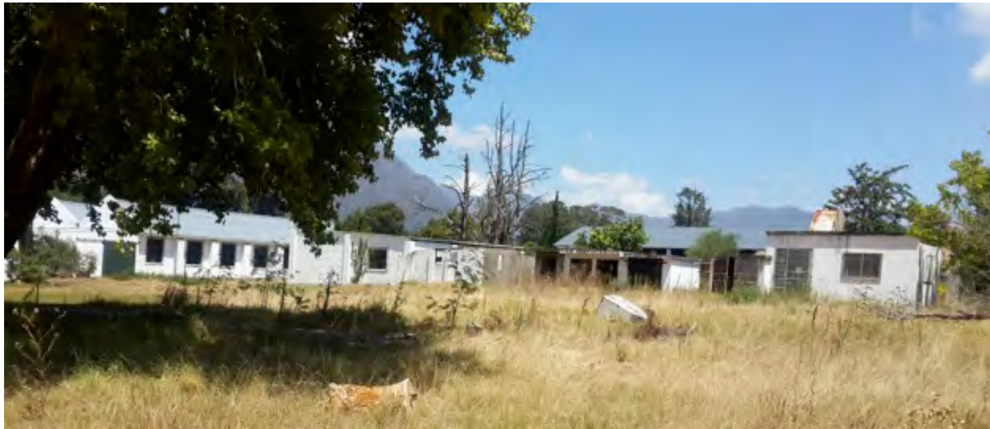
Photos 7-8: Pack shed constructed between 1953 and 1966. Associated with the diversification of the fruit industry on Rhodes Fruit Farms during the mid 20th century.
